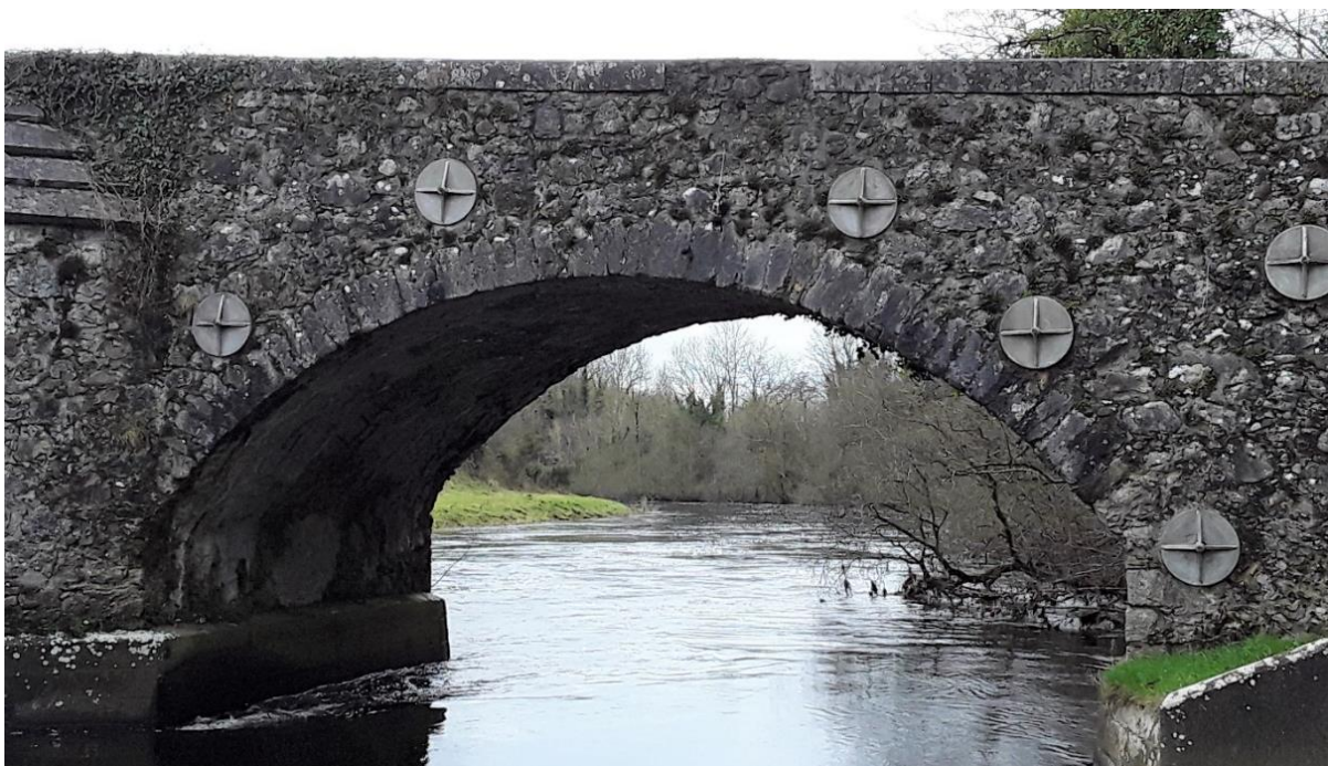
Photo 15: Newcastle Bridge after strengthening work
