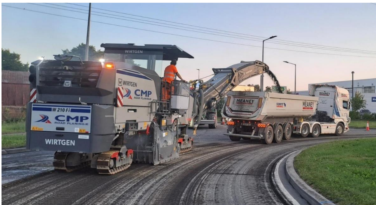
Photo 13: Recycling of road materials on Longford Town N4 bypass
