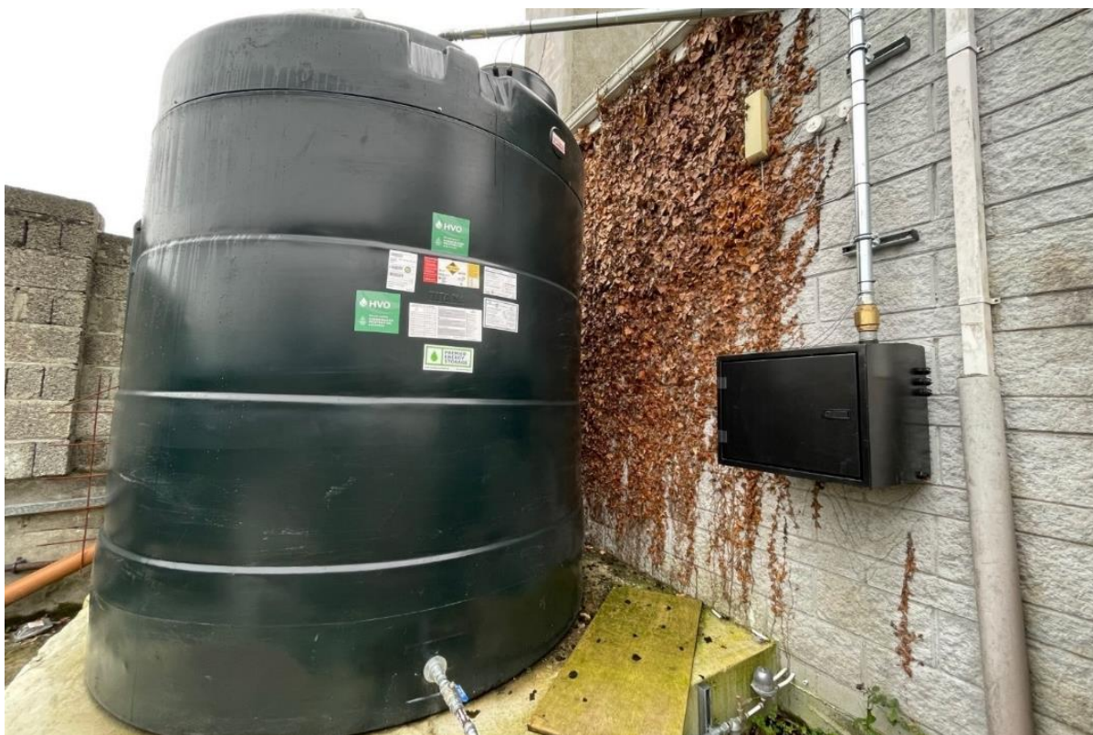
Photo 25: New HVO tank as Áras an Chontae
