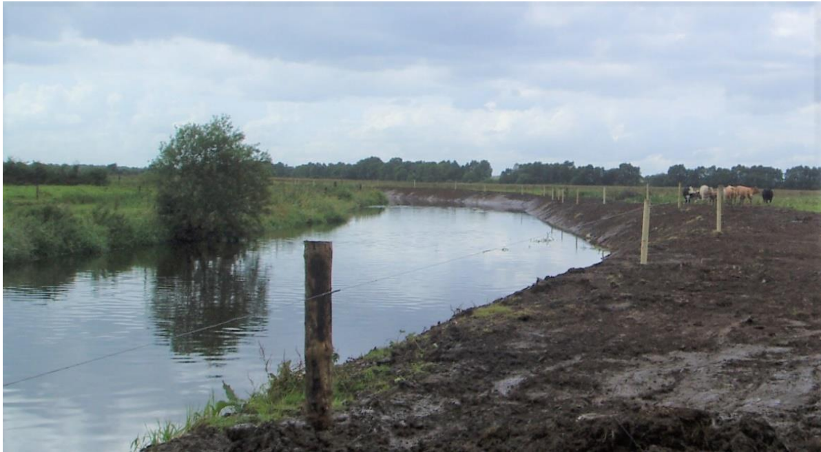
Photo 19: Channel cleaning on the River Camlin
