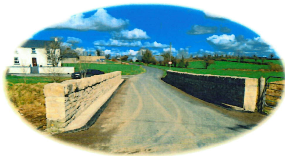
Image of Ballyduffy Bridge Works – 2023
