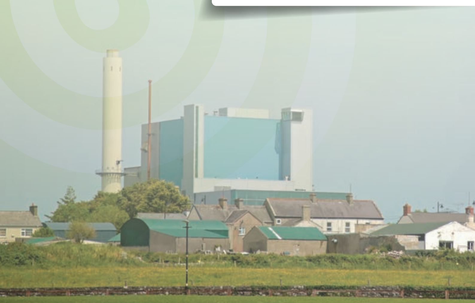
The former Lanesborough Power Station
