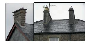
Chimneys are important visual features in a dwelling and should be located on the ridge line where possible, particularly in the case of hipped roofs, or located to the rear. The traditional style chimneys illustrated above are all substantial structures and read as strong design elements. Thin, insubstantial chimney structures should be avoided.
