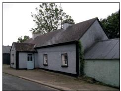
The roof and roofing material is an important element in the visual impression of a dwelling, particularly in terms of how the bulk of the building is articulated. Traditional rural built forms were long in plan and appearance. Pitches are usually set between 40°-45°.
