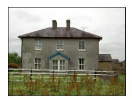
Hipped roofs can be utilised to reduce the visual bulk of square plan houses, an effect that is negated where chimneys are placed at either gable end.
