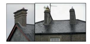
Chimneys are important visual features in a dwelling and should be located on the ridge line where possible, particularly in the case of hipped roofs, or located to the rear. The traditional style chimneys illustrated above are all substantial structures and read as strong design elements. Thin, insubstantial chimney structures should be avoided.
