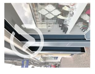
Fig. 27. Roller shutter guides should be integrated into the shop front in rare cases where externally installed roller shutters are permitted.
