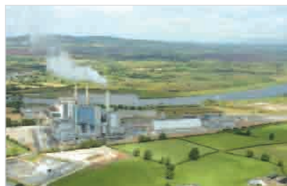
Lough Ree Power Station, Lanesboro
