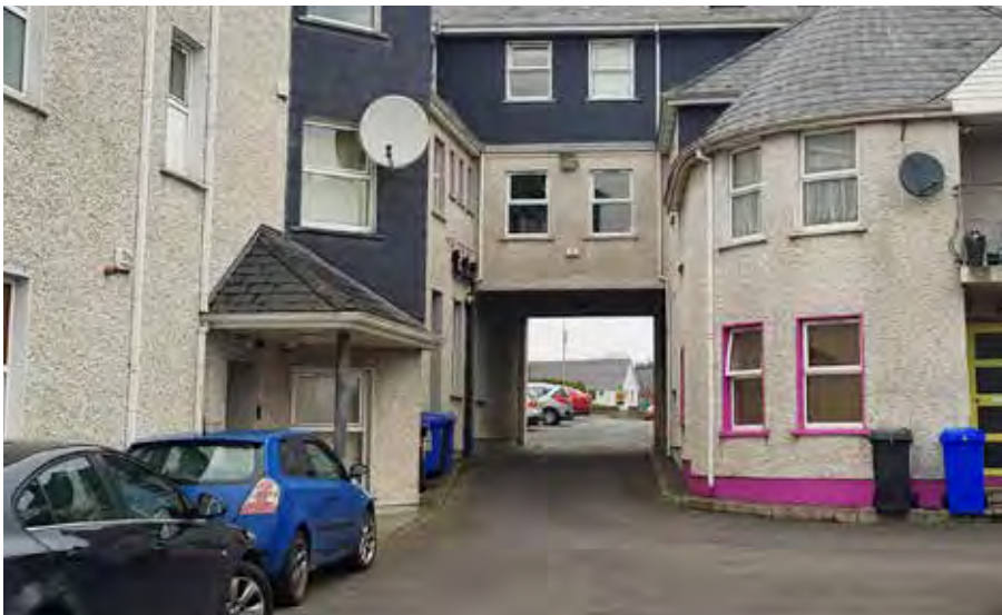
Car dominated streetscape with lack of safe pedestrian movement and access
