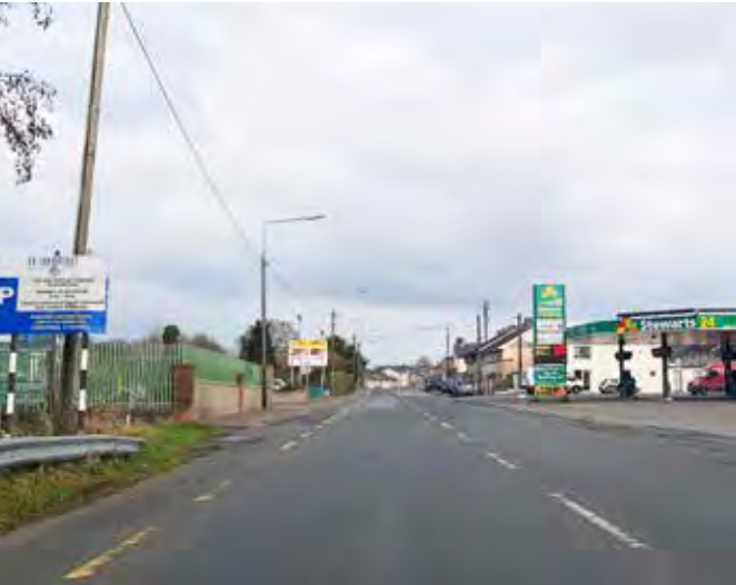
Weak primary gateway along Connaught Road
