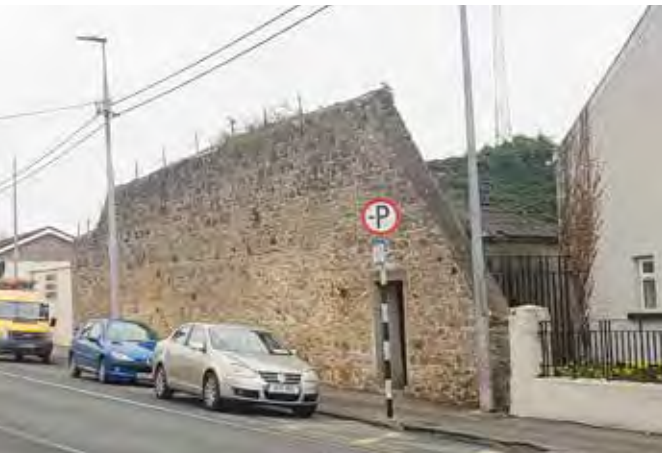
Protected boundary wall on Church Street
