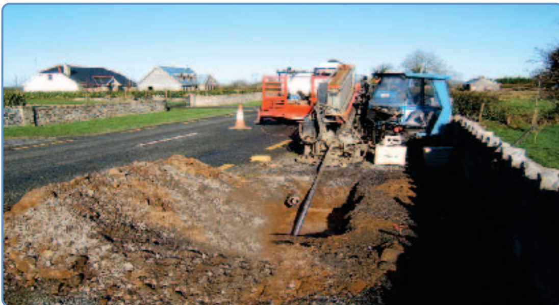
Ardagh Group Water Scheme: Directional drilling
