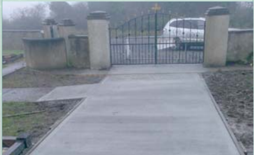
New Wheelchair Accessible footpaths at Barraghmore Cemetery
