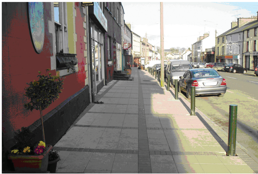
Environmental Improvement works in Granard
