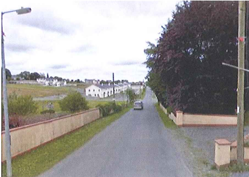
View overlooking bridge from south
