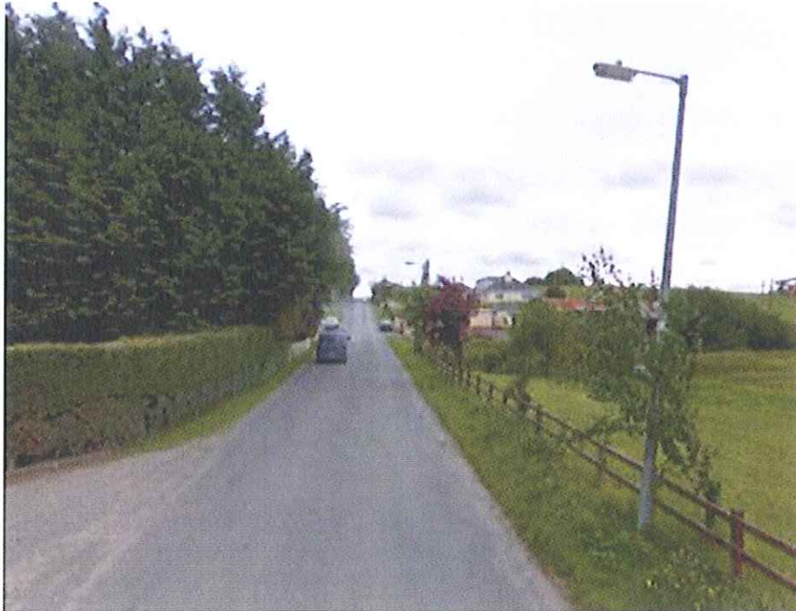
View overlooking bridge from north
