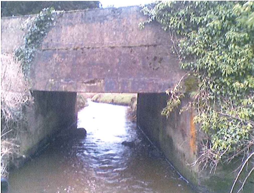
Upstream elevation of bridge
