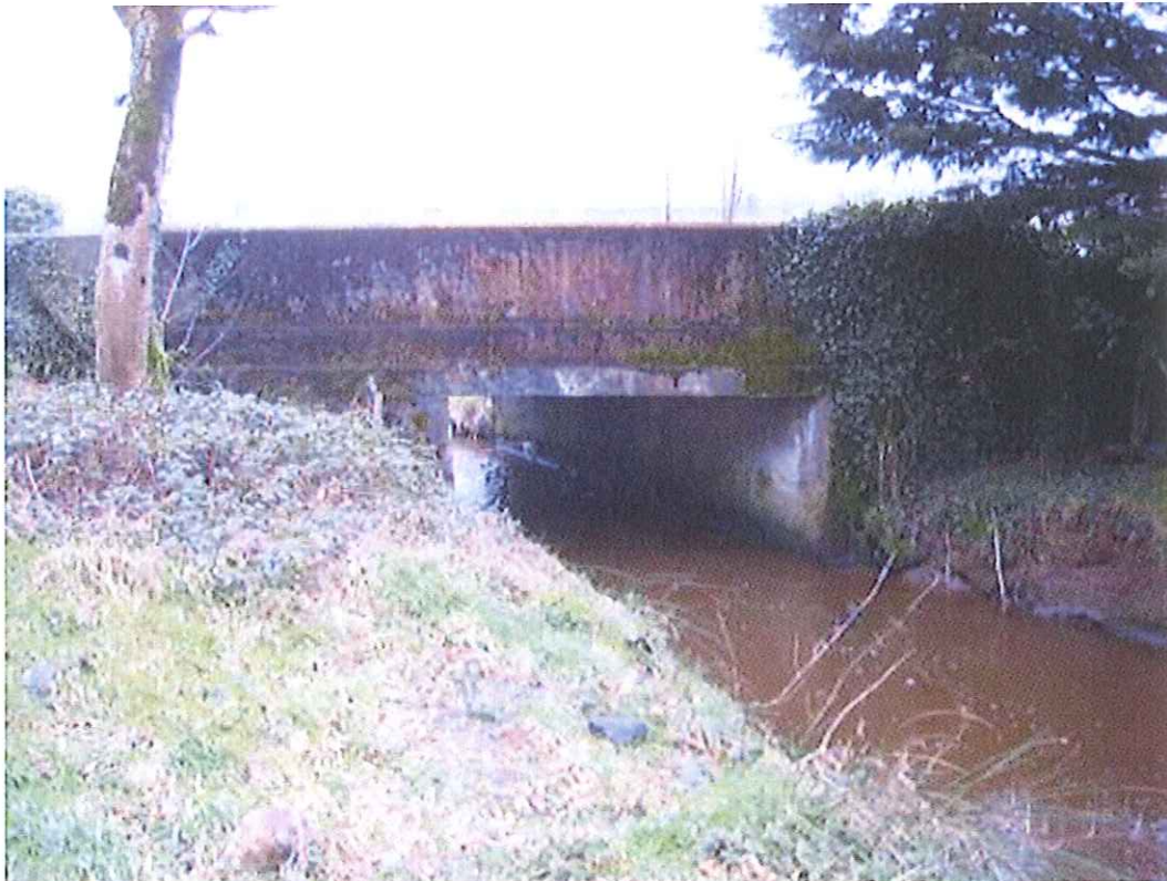
Downstream elevation of bridge
