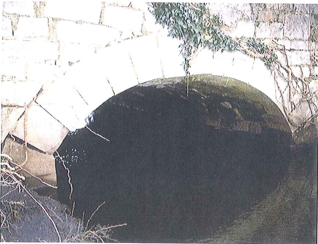
View of downstream elevation
