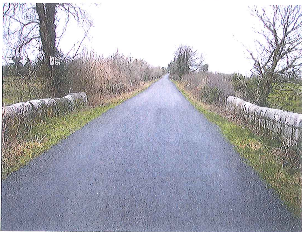
View overlooking bridge from west
