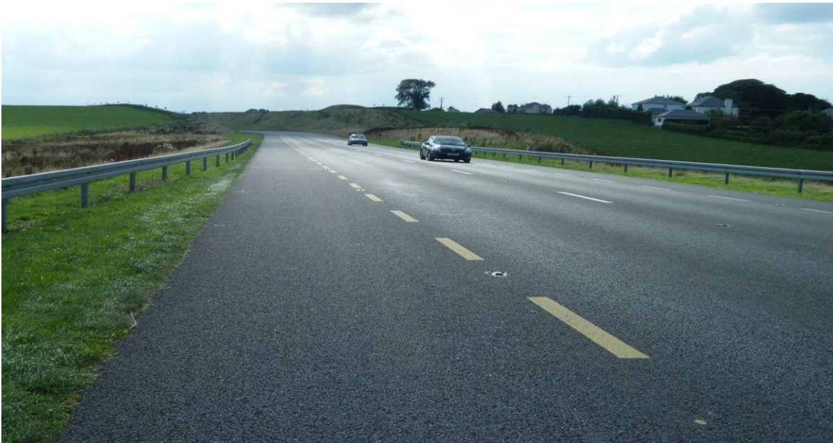
N5 Longford Bypass
