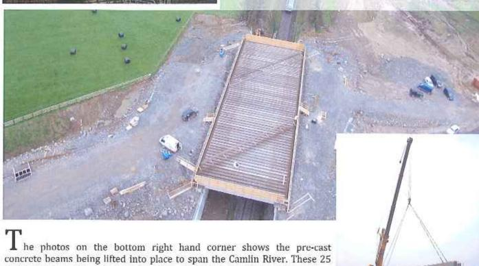
concrete beams being lifted into place to span the Camlin River. These 25 metre long beams were produced in Banagher in Offaly and weigh a staggering 48 tonnes each.
