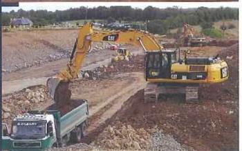
Work has also been progressing steadily on the construction of the roundabouts particularly at the N4 Sligo Road. As you will see from the photo on the cover page of the newsletter the roundabout has been shaped in its totality. The installation of gullies, manholes and utility ducting will be completed in the foreseeable days.
