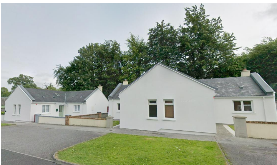
Photo 4 Newly energy retrofitted houses at Abbeycartron Lane.
