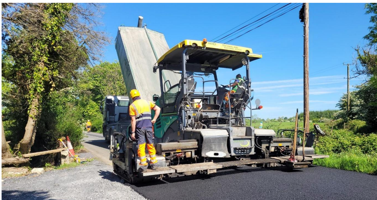
Photo 9 Laying warm mix macadam in North Longford
