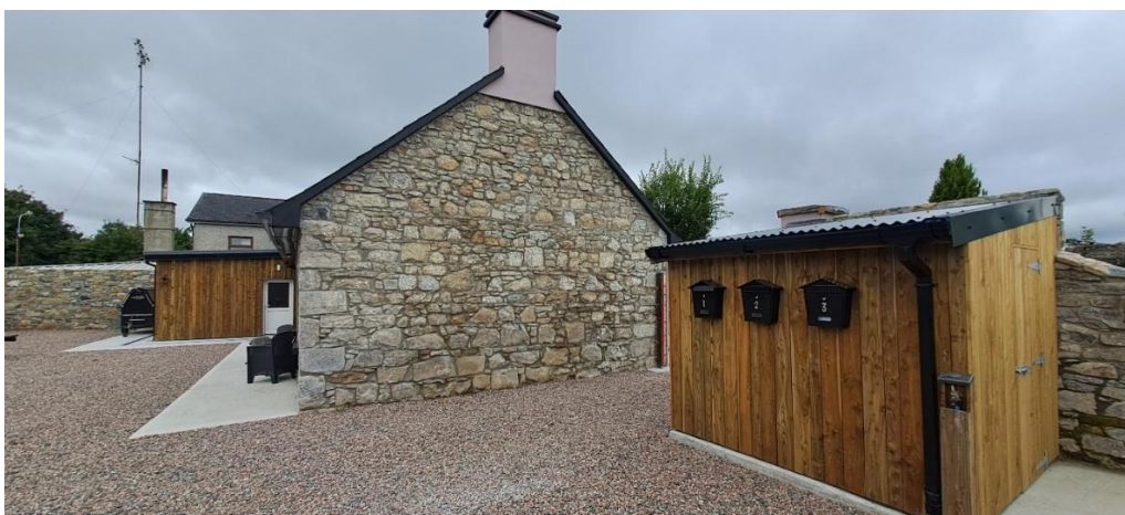
Photos 5 & 6 Vacant Property Refurbishment
