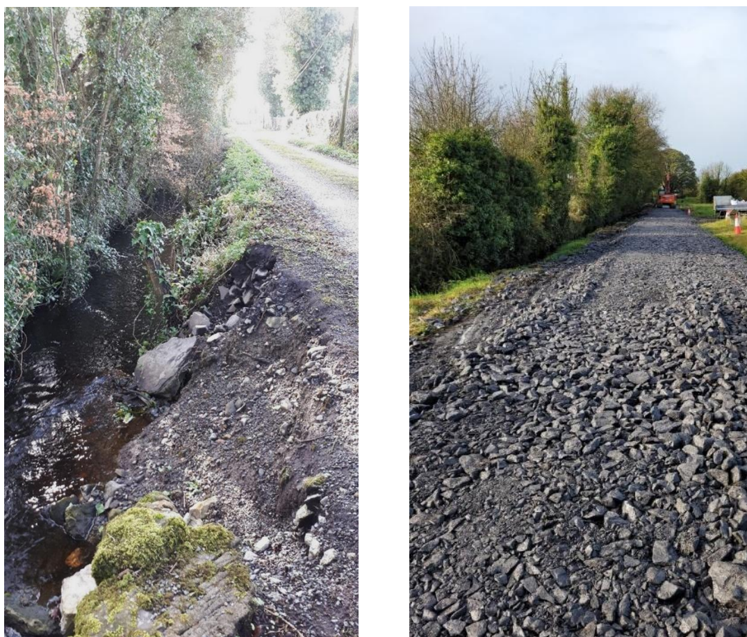
Photos 7 & 8 Ringowney Lane, before and during construction.
