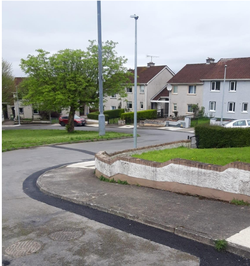
Photo 12 Upgraded public lighting at Pauric Colum Heights showing new cabling.
