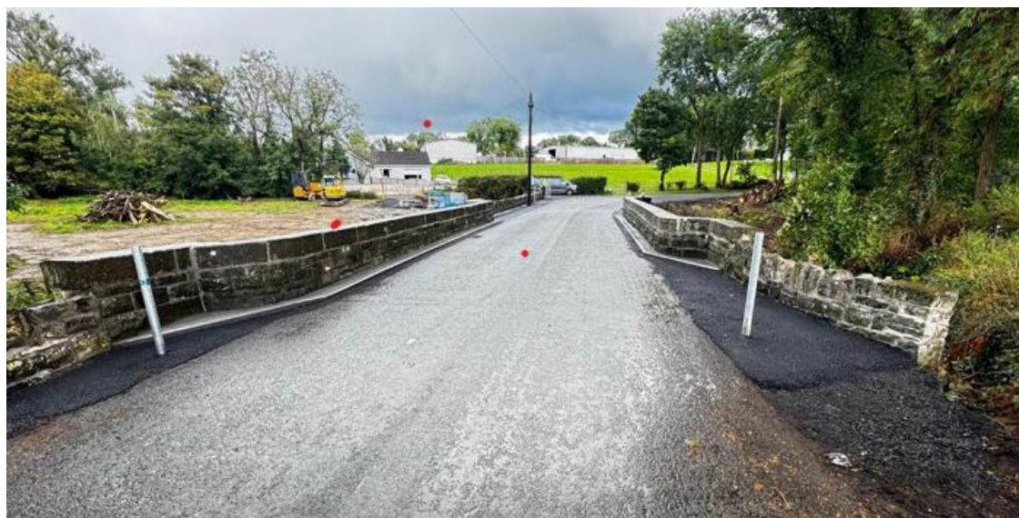
Photo 11 Kilnacarrow Bridge after rehabilitation works in 2025
