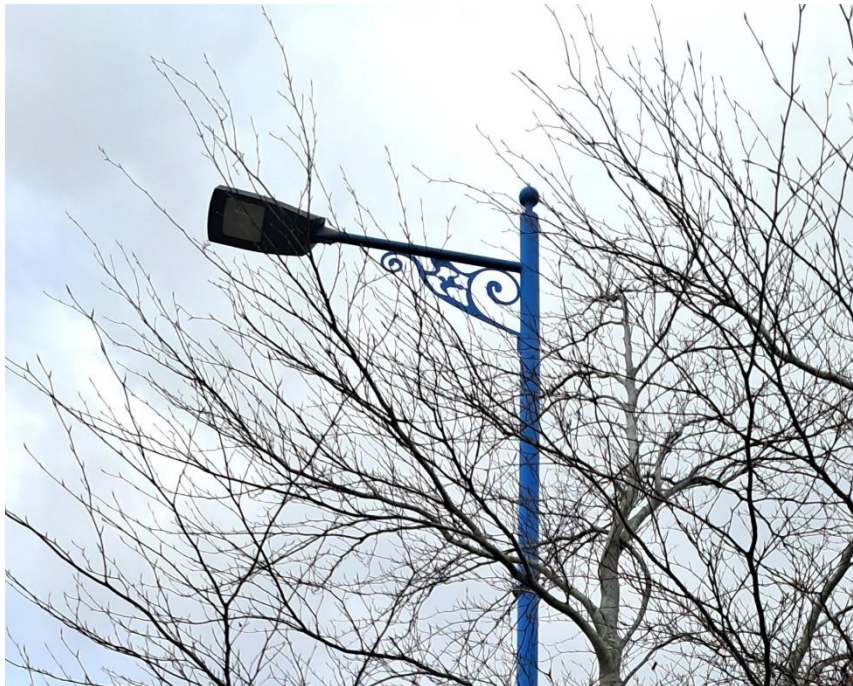
Photo – new LED light installed in Newtowncashel
