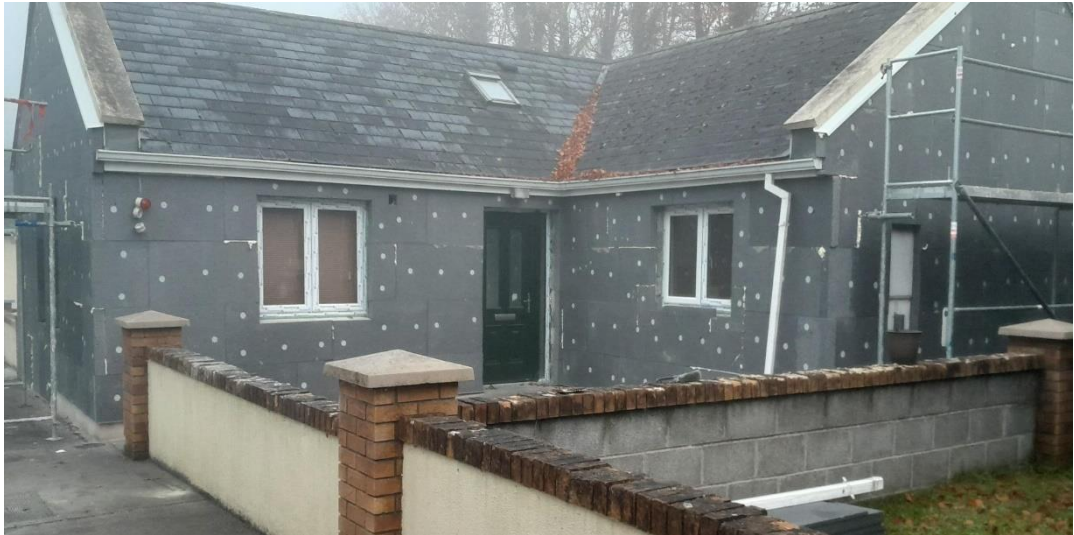
Photo – House retrofit Fairgreen View, County Longford.
