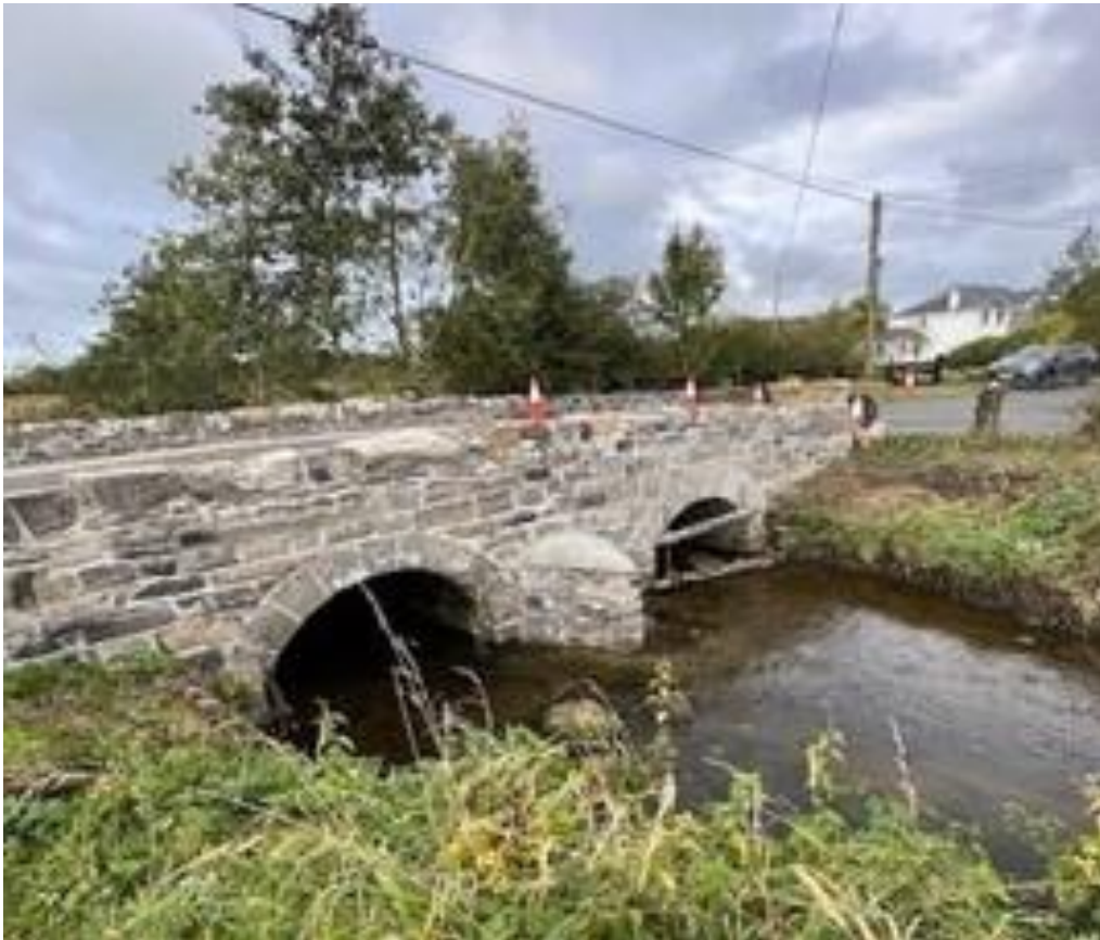
Photo – rehabilitated bridge at Liscahill-Gneeve 2024
