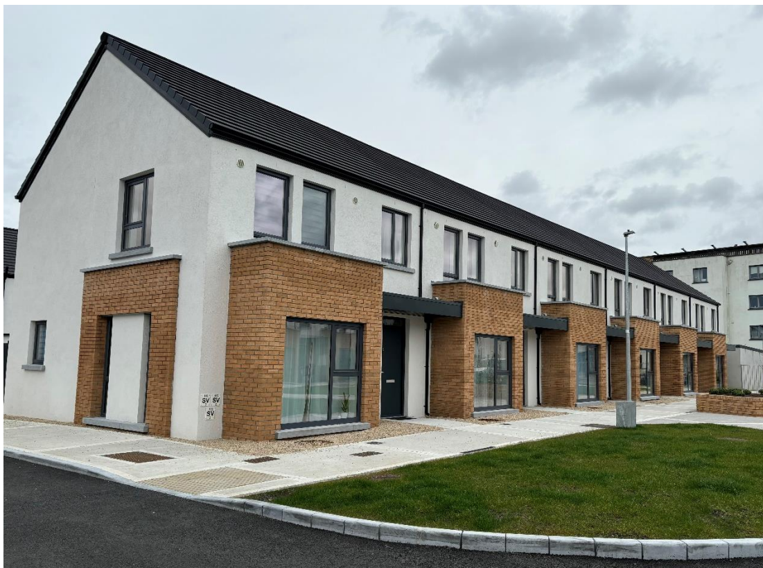
Photo – New local authority houses on Connaught Road, Longford
