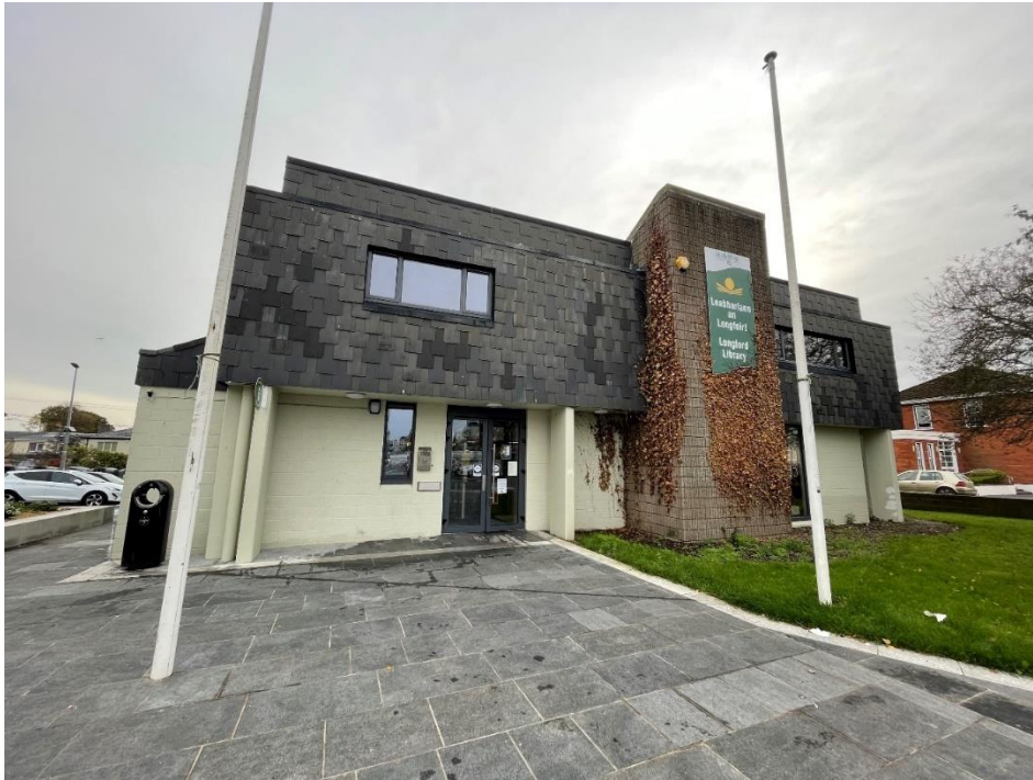
Photo 24 Longford Library after doors, windows, and internal lighting upgrades
