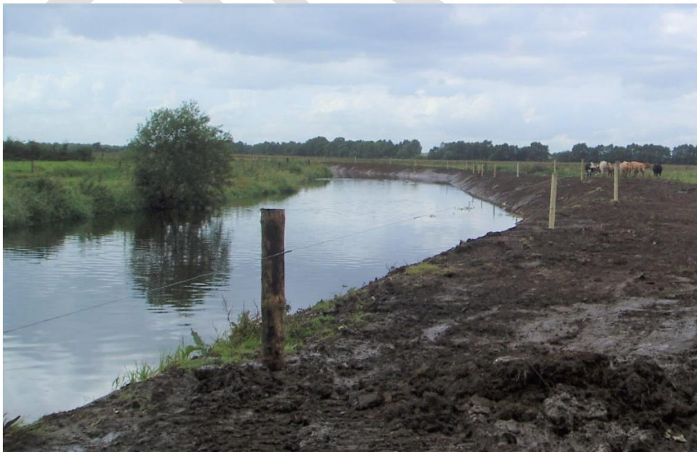
Photo 19 Channel Cleaning on the River Camlin
