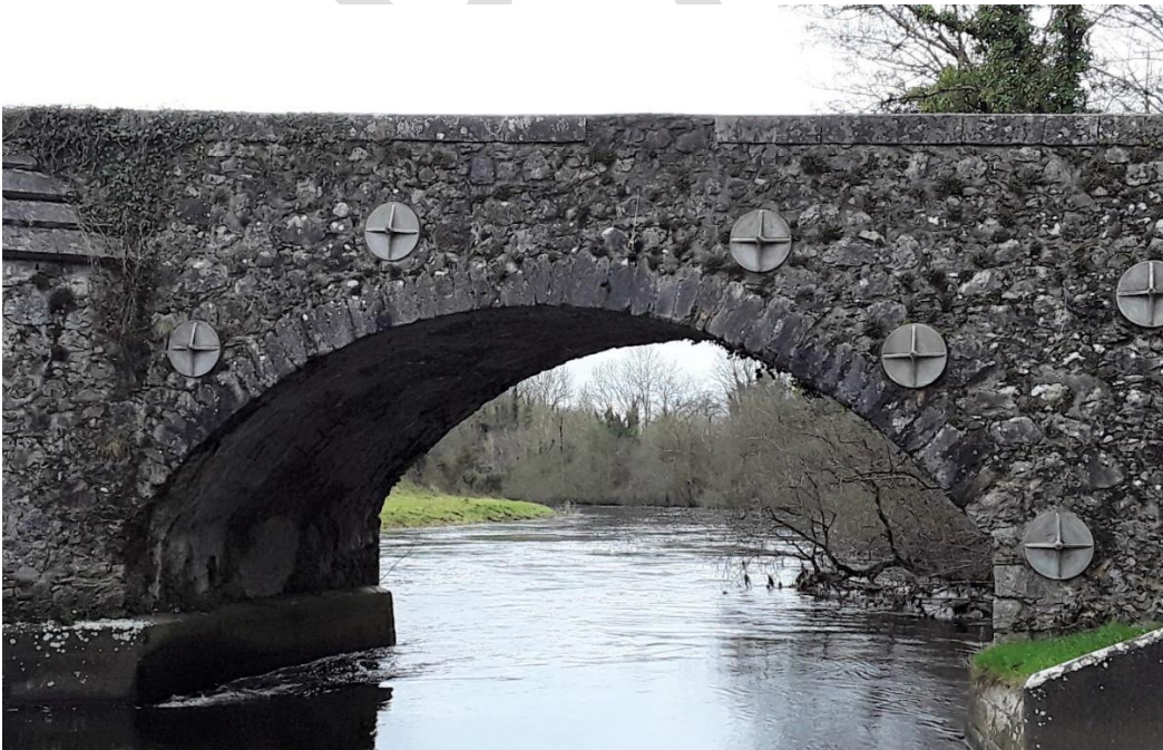
Photo 15 Newcastle Bridge after strengthening work
