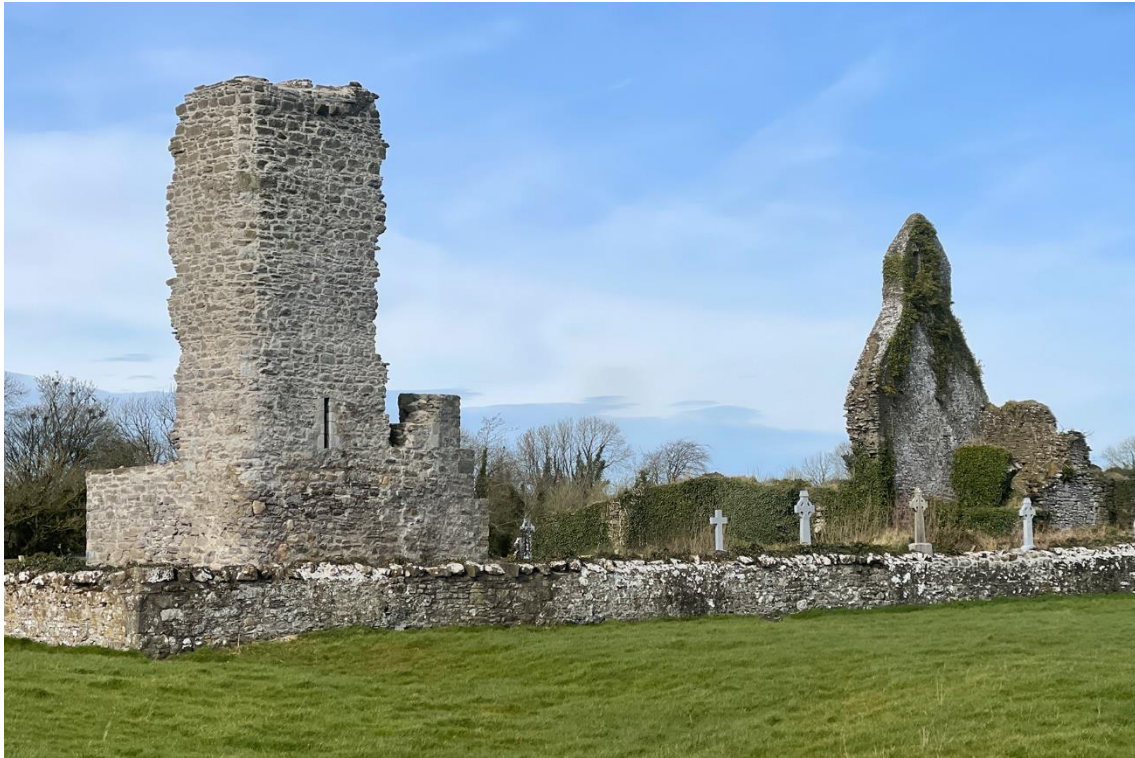
Photo 9 Abbeysrule Abbey following conservation work in 2021
