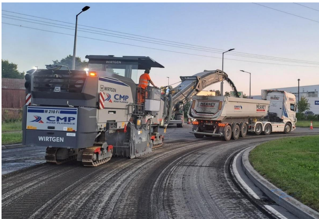
Photo 13 Recycling of road materials on Longford Town N4 bypass
