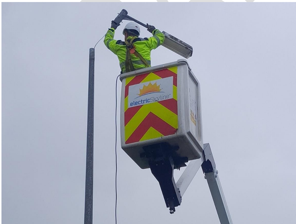
Photo 12 Public Lighting upgrade works at Gleann Riada, Longford
