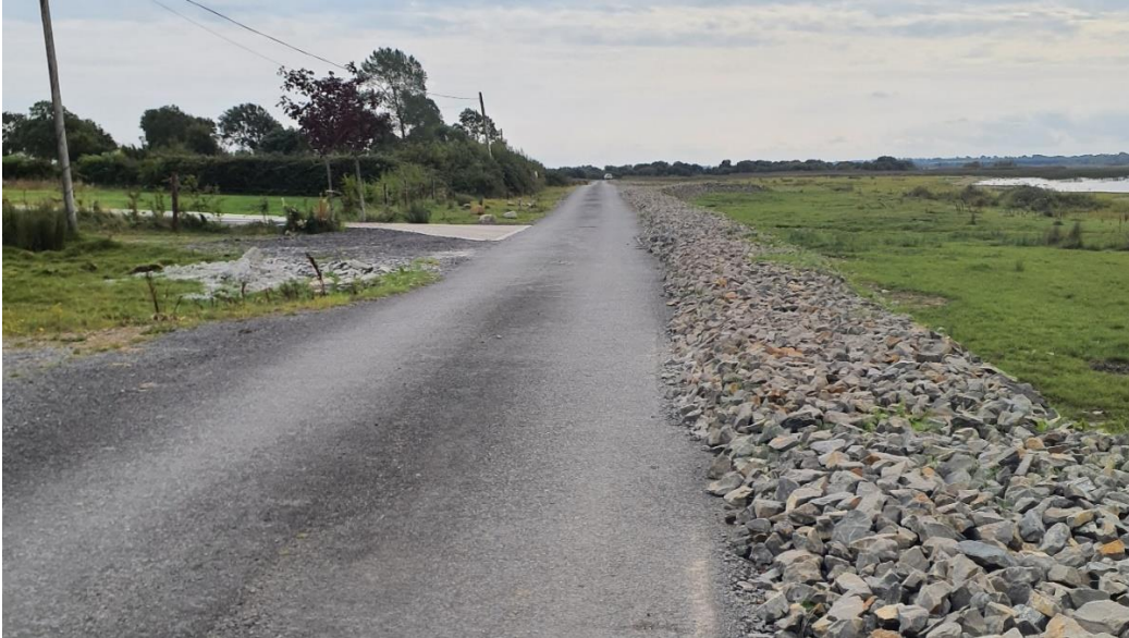
Photo 14 Saints Island Road adaptation works
