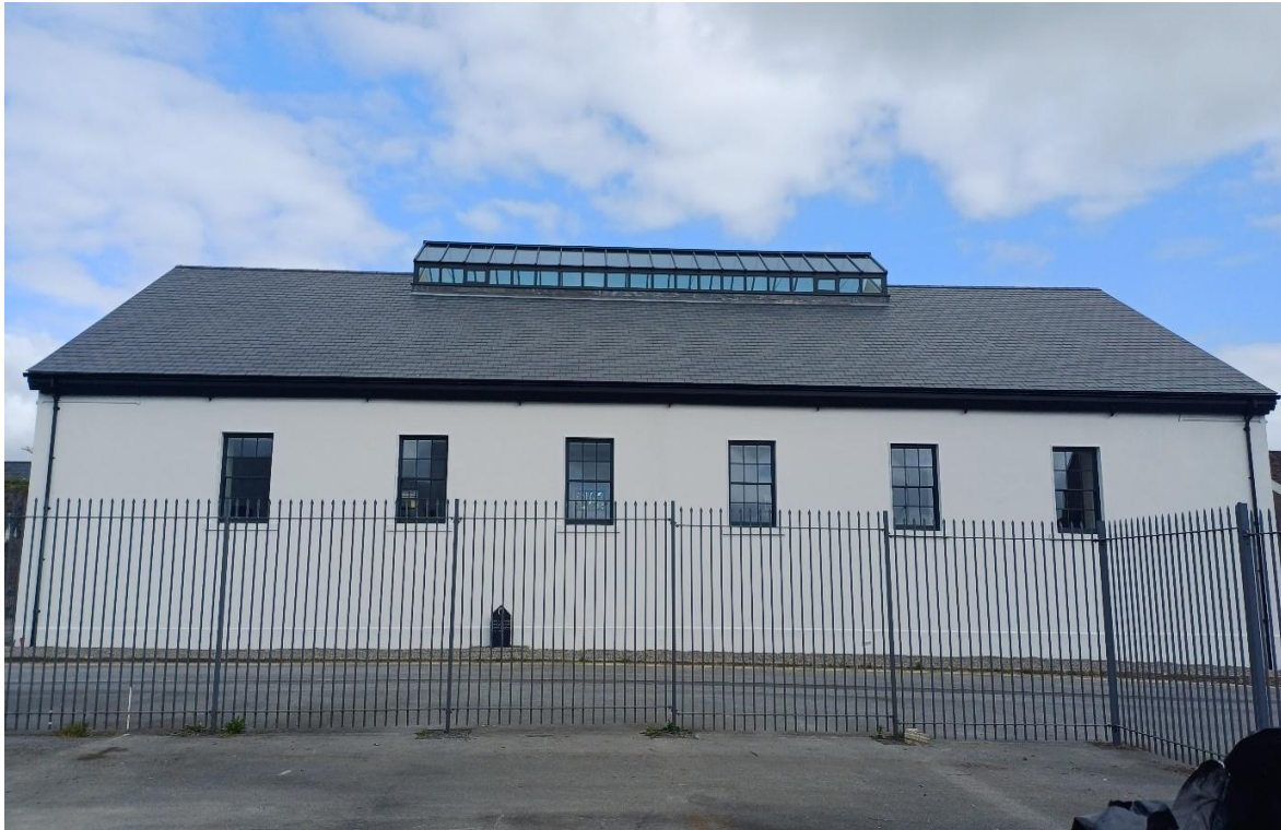
LWETB Refurbished building at Connolly Barracks Site Longford Town
