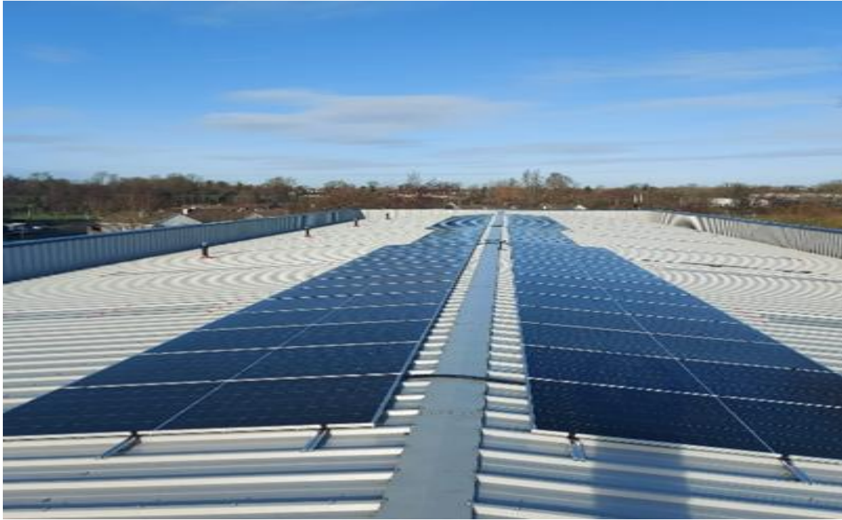
Installation of new solar panels on the roof of Longford Athletics Club funded under the CCAP.
