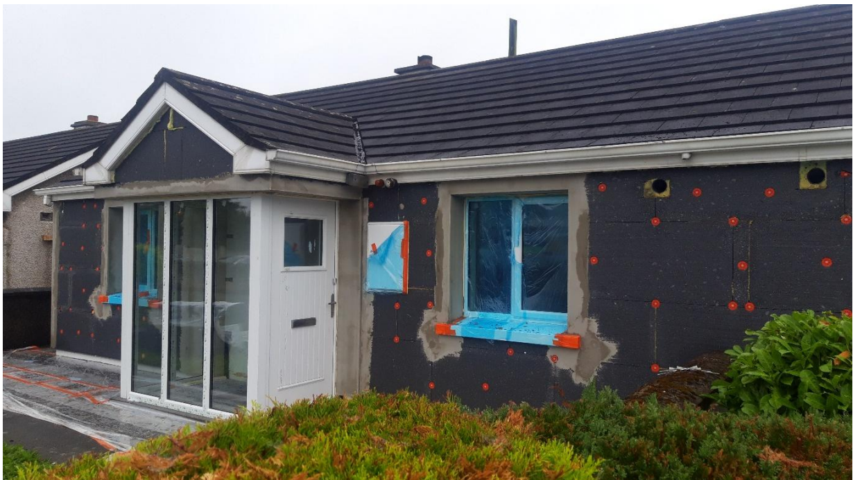
Housing Retrofit at Athlone Road, Longford Town.
