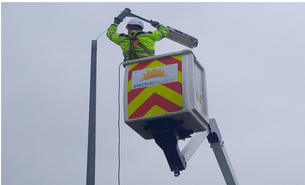
Public lighting being upgraded at Gleann Riada, Longford Town.
