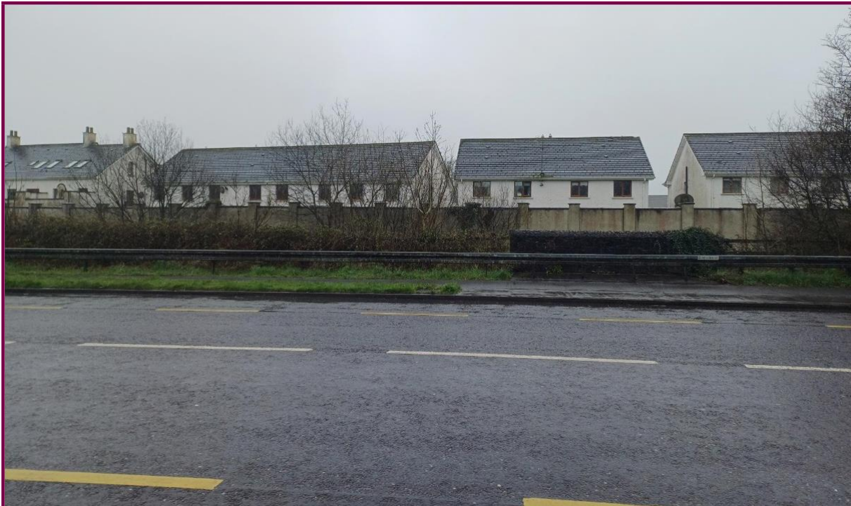
Figure 20: View from N4 to PIA (Mostrim Oaks), photograph March 2024. Showing 3m high boundary wall constructed as noise barrier / noise mitigation (condition of planning permission 04-1060 )
