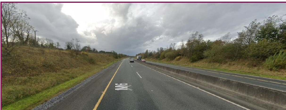
Figure 36: Example of a road cutting, where the cutting provides noise screening, similar to an earth berm (Source: Google Maps, M6 Street View).
