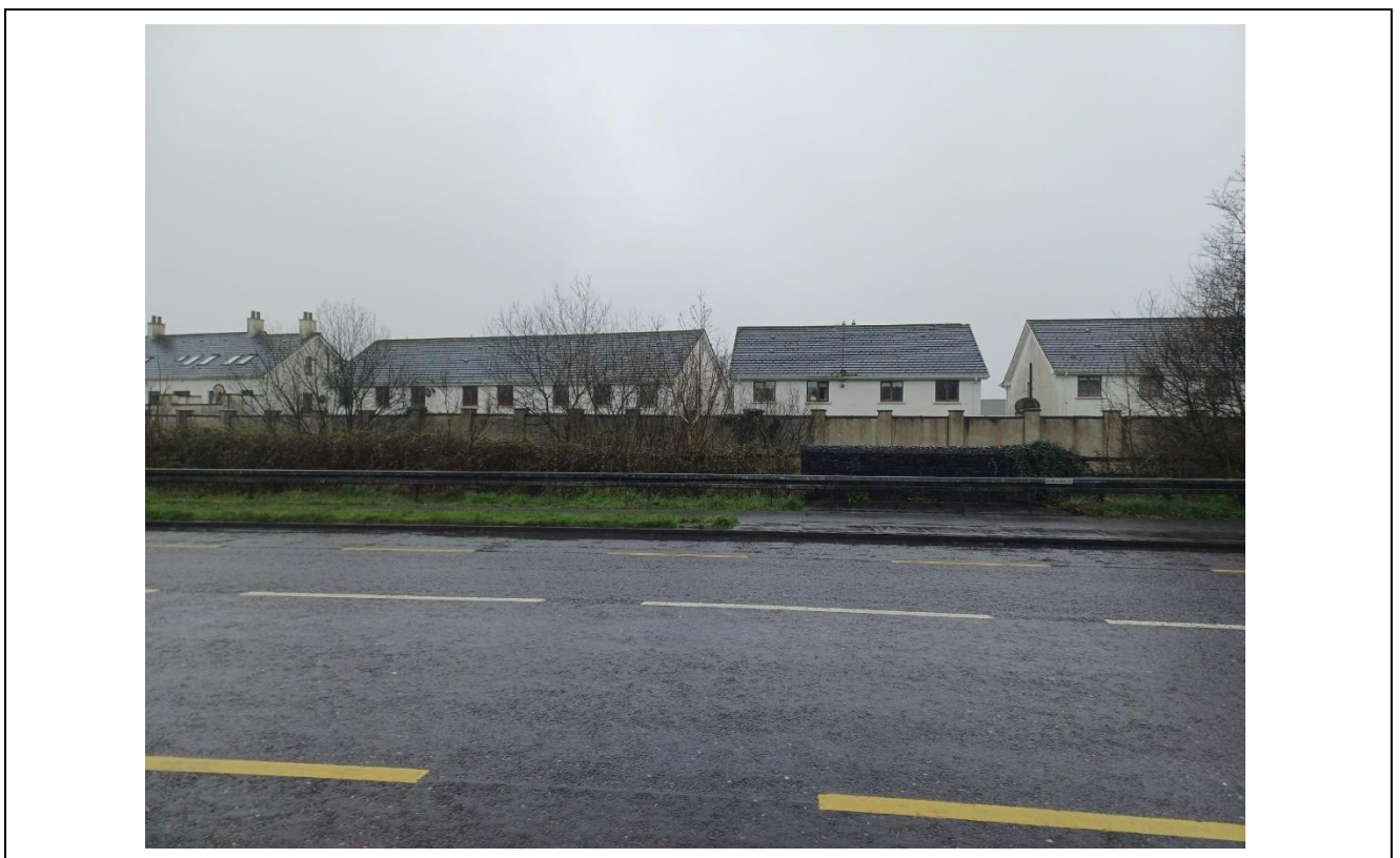
Figure 21: View from N4 to PIA (Mostrim Oaks), photograph March 2024. Showing 3m high boundary wall constructed as noise barrier / noise mitigation (condition of planning permission 04-1060 )
