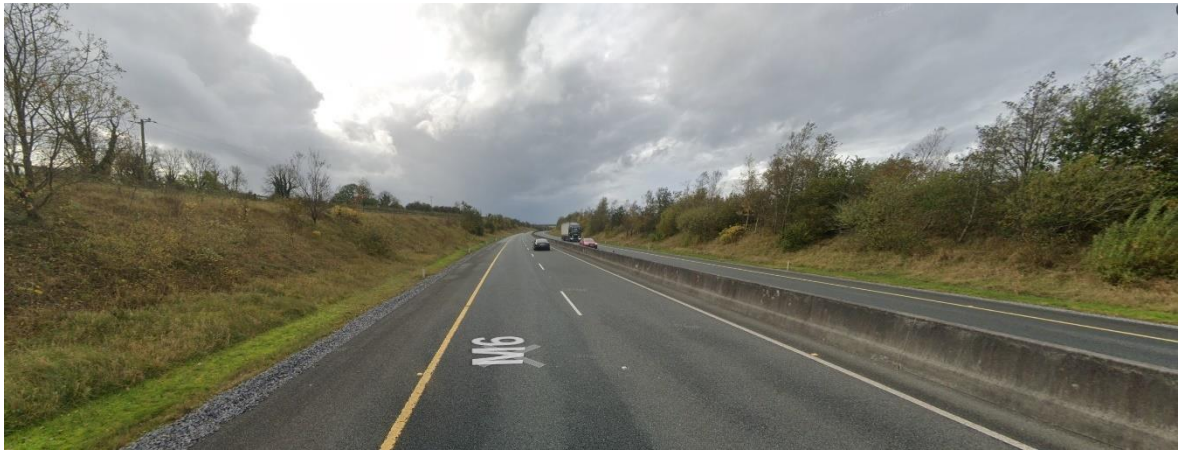
Figure 38: Example of a road cutting, where the cutting provides noise screening, similar to a earth berm (Source: Google Maps, M6 Street View).
