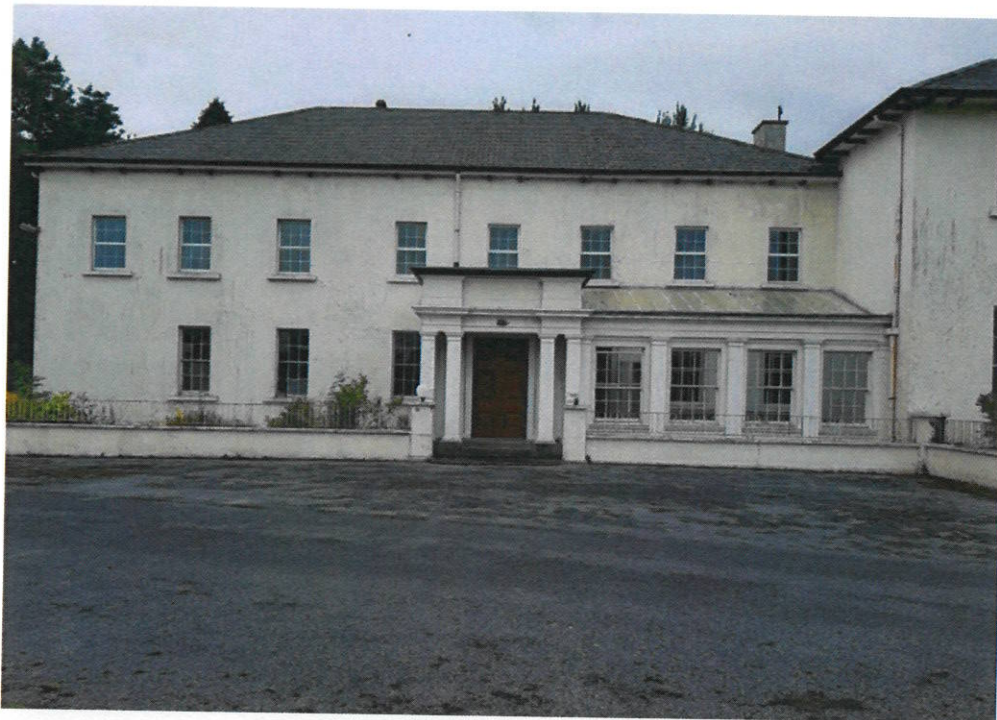
Exterior of the front of Ardagh House
