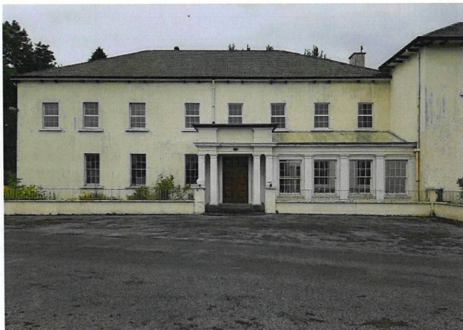
Exterior of the front of Ardagh House
