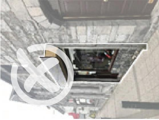
**Fig. 25.** Projecting roller shutter boxes will not be permitted.
