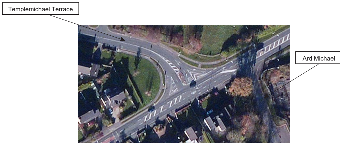
Figure 3.1: Exiting N63 Major's Well Junction
