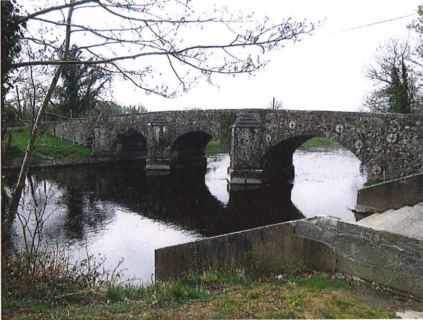
Newcastle Bridge and concrete steps descending to river edge
