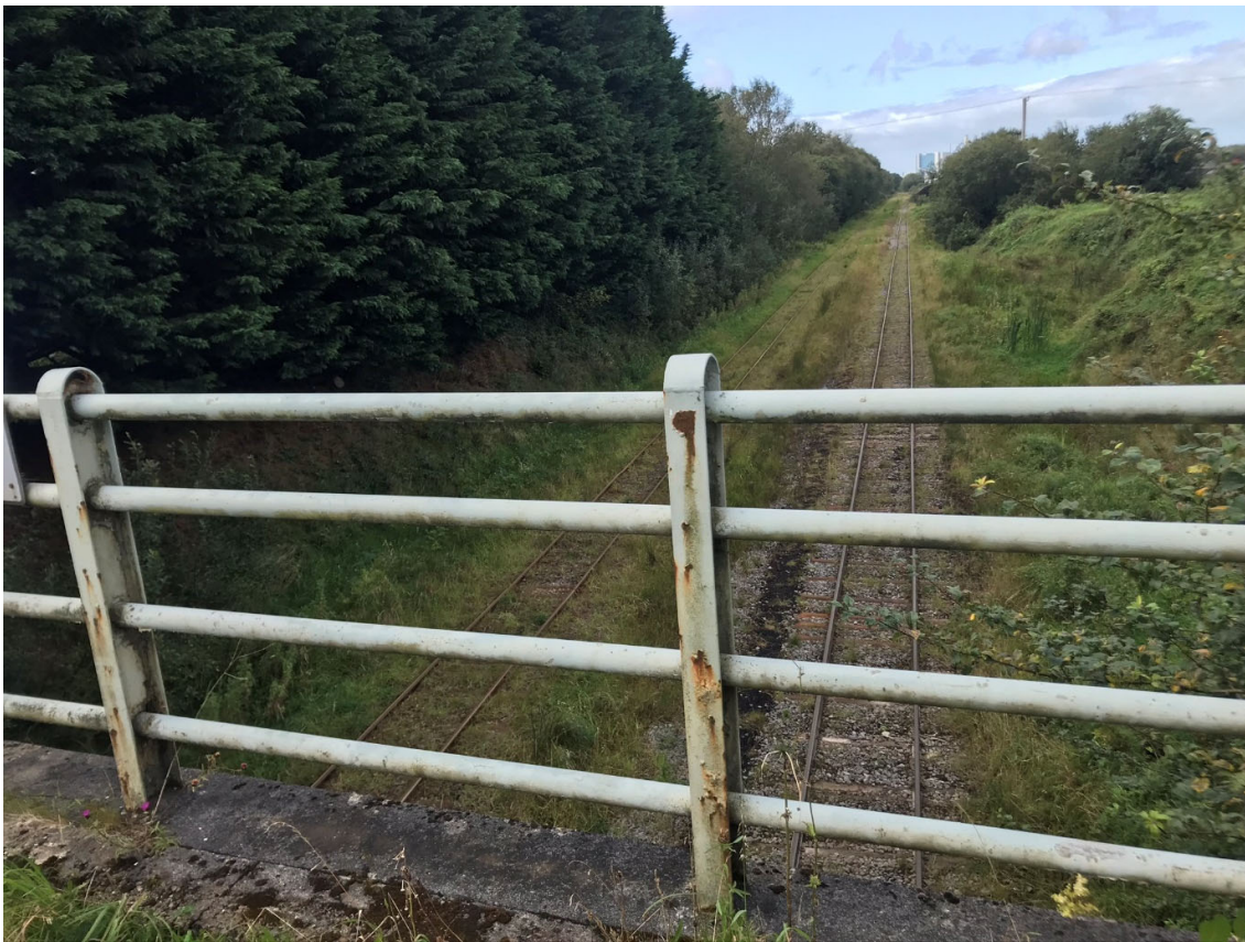
Figure 2: Decommissioned Bord Na Mona Industrial Railway
