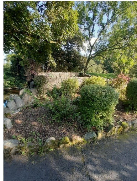
Existing Stone Abutment on the East
