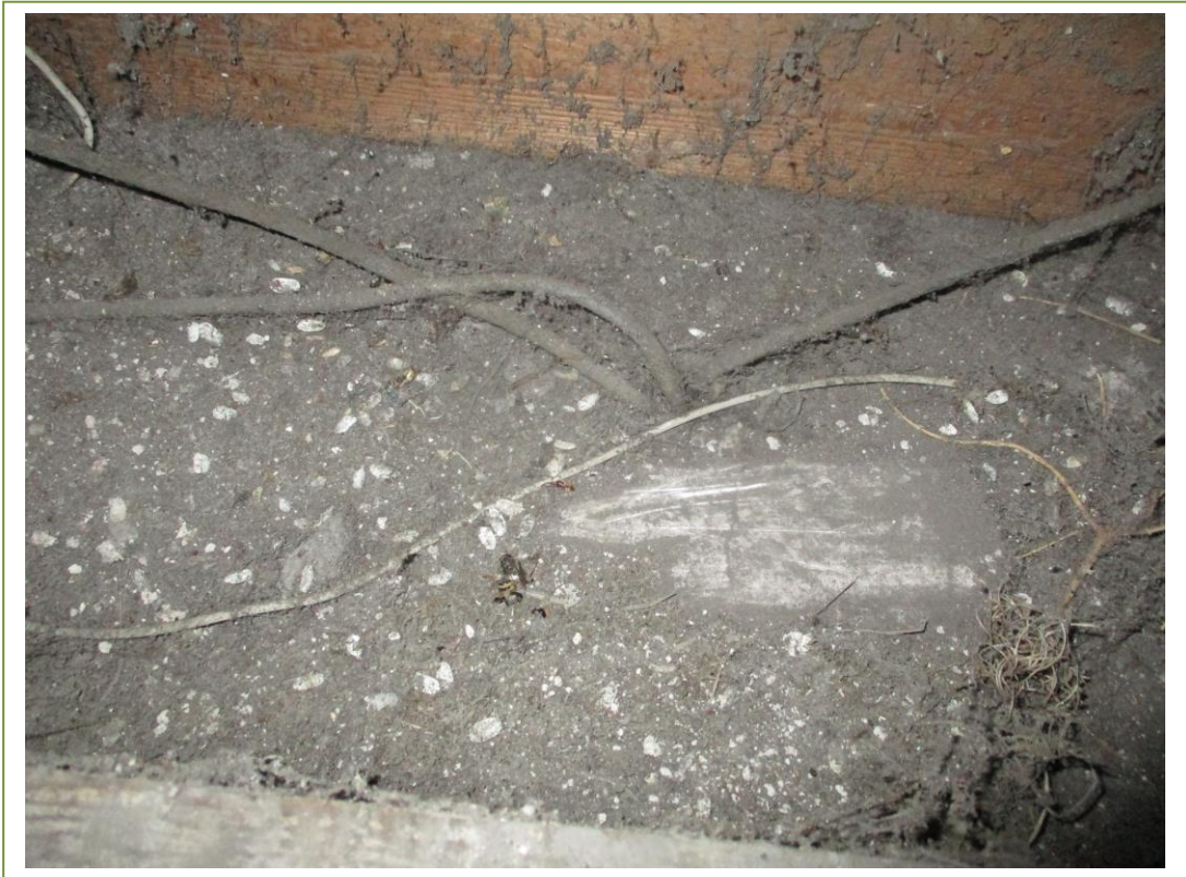
Plasterboard on the ceilings
