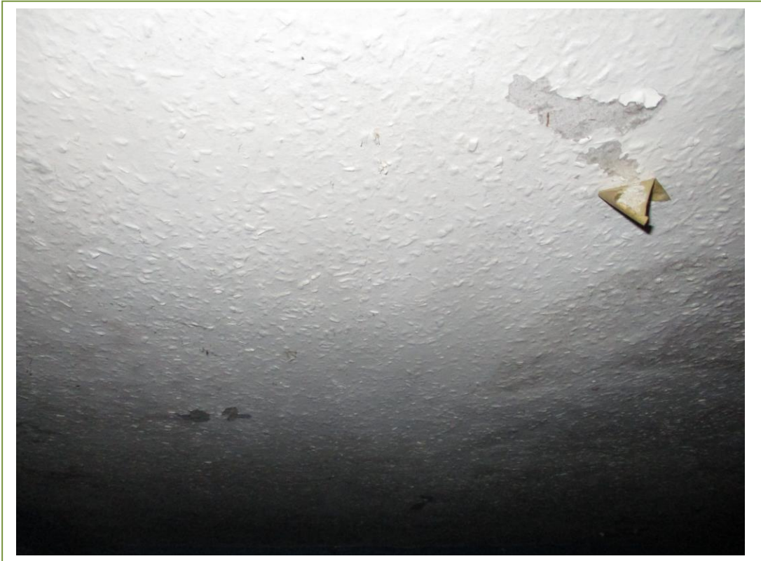
Woodchip paper on the kitchen ceiling
