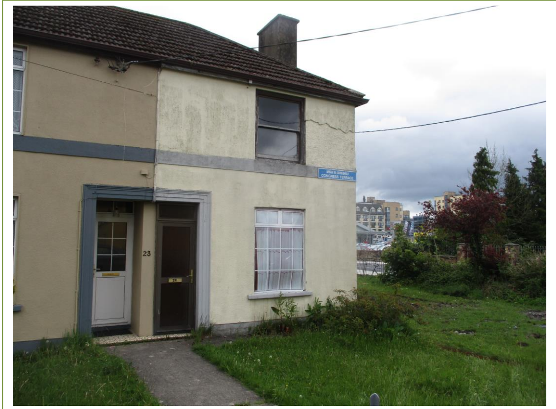
Concrete tiles on the roof of the house
