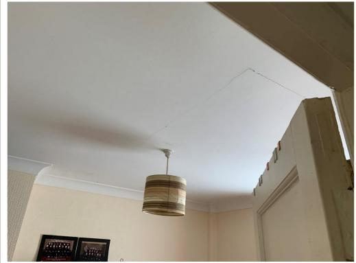
Cracking in the ceiling of the first floor bedroom to the front of the property.
