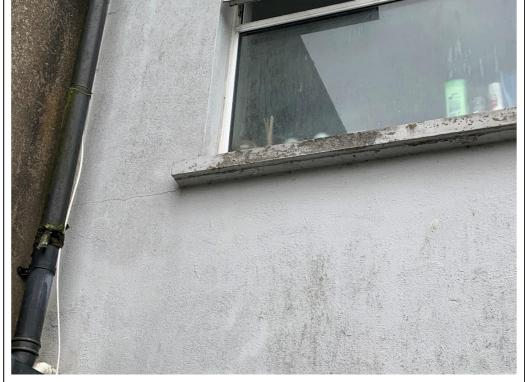
Horizontal cracking at cill level of first floor bathroom window.
