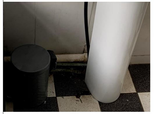
Leaky pipe work present in the first floor bathroom, which may contribute to the staining to party wall at ground floor level.
