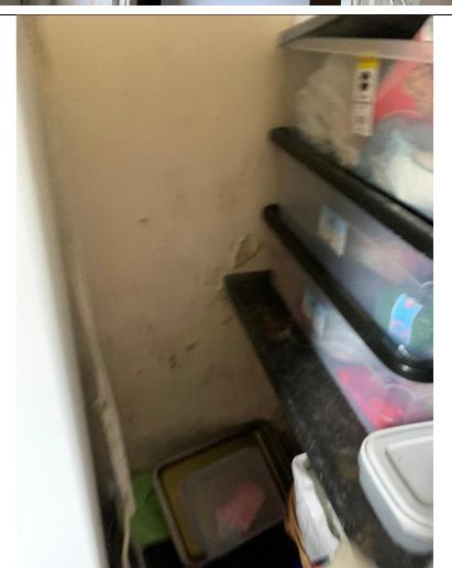
Low level damp and flaking paint indicates rising damp present along the party wall of no 23 and no 24.
