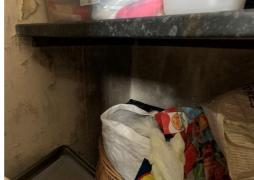
Further indication of damp present in the property, the use of a washing machine and tumble dryies in this area would also be a contributing factor due to lack of ventilation.
