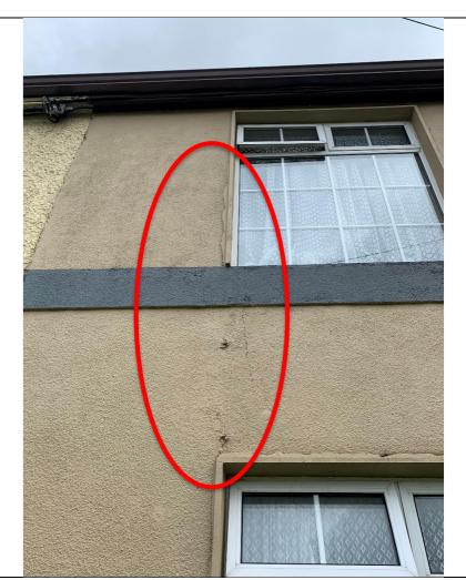
Vertical cracking in the plastered render between the ground floor and first floor windows.
