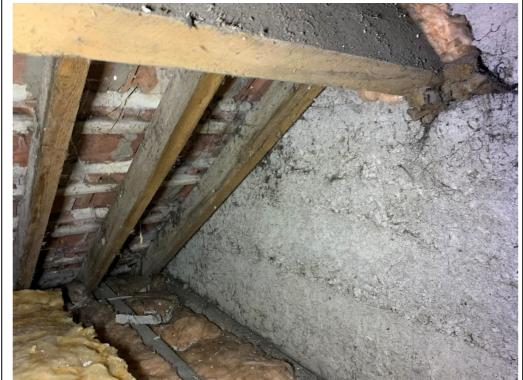
No evidence of fire stopping between properties.
