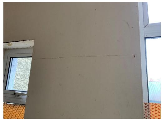
Horizontal crack between windows in kitchen area.
