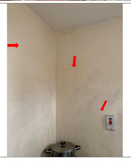
Kitchen located to rear of property. Diagonal crack staggering between two walls
