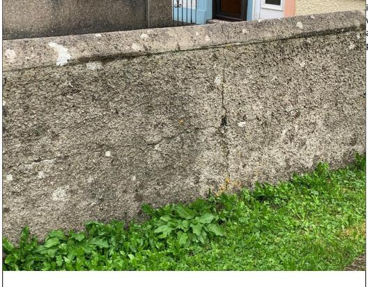
Multiple cracking in the boundary wall to the front and side of the property.
