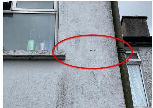
Horizontal cracking on RHS of first floor bathroom window at cill level,
