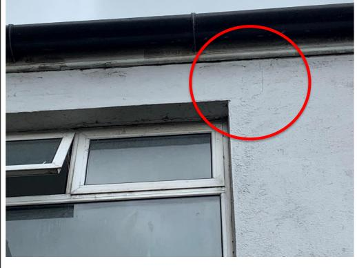
Diagonal crack to RHS of first floor window head.
