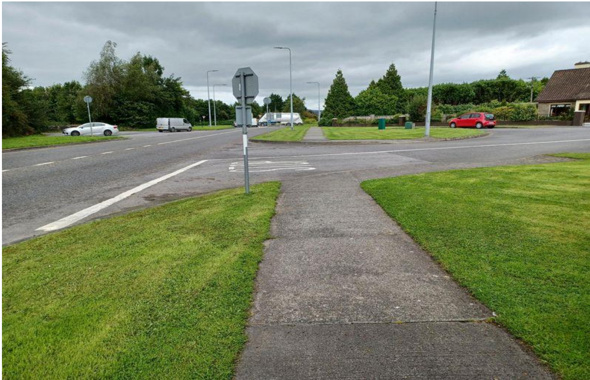
View of junction at entrance to The Laurels Estate. It is proposed to tighten this junction to a 3m radius.
