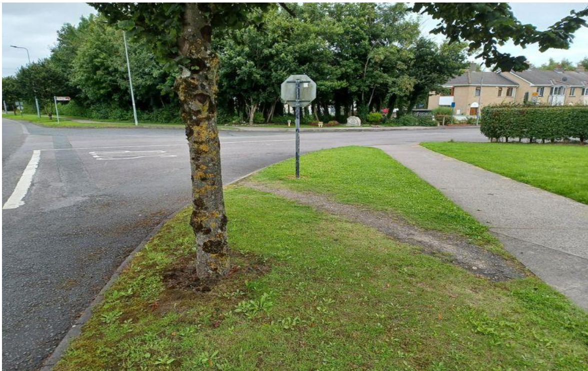
View of junction at entry to St.Emers Estate and one way entry to St. Emers N.S. It is proposed to tighten this very wide junction to a 6m radius.
