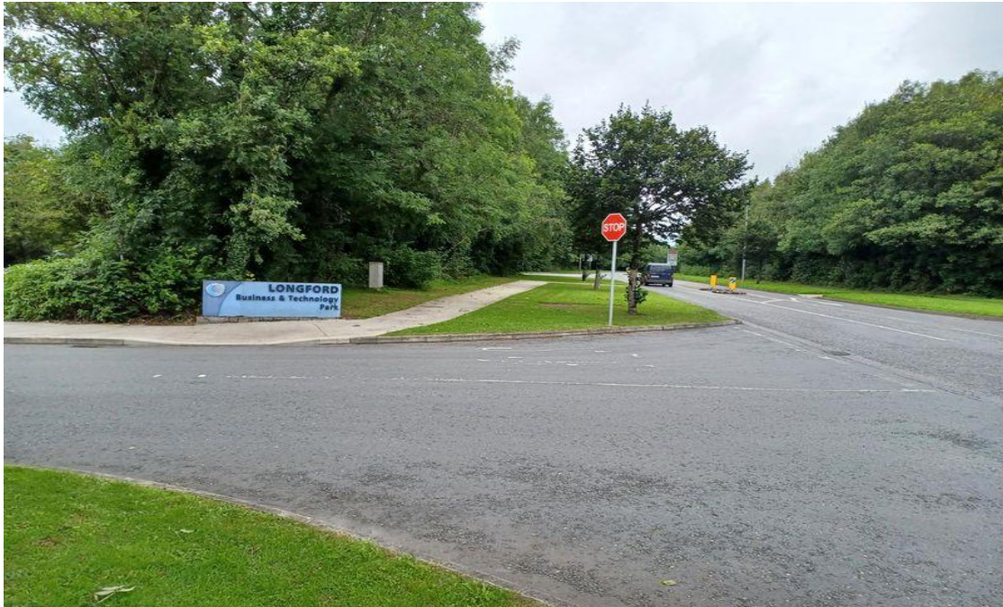
View at wide junction at entrance to Longford Business and Technology Park. It is proposed to tighten this wide junction to a 9m radius.
