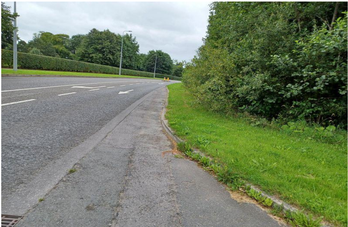
Image shows View towards Major Wells Road (Town Centre) from RHS @junctions. It is proposed to reinstate the old kerbline when Junction Tightening in this location.
