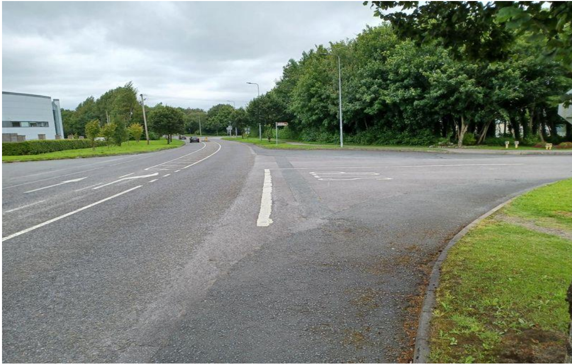
Another image showing this very wide junction at entry to St. Emers Estate and National School
