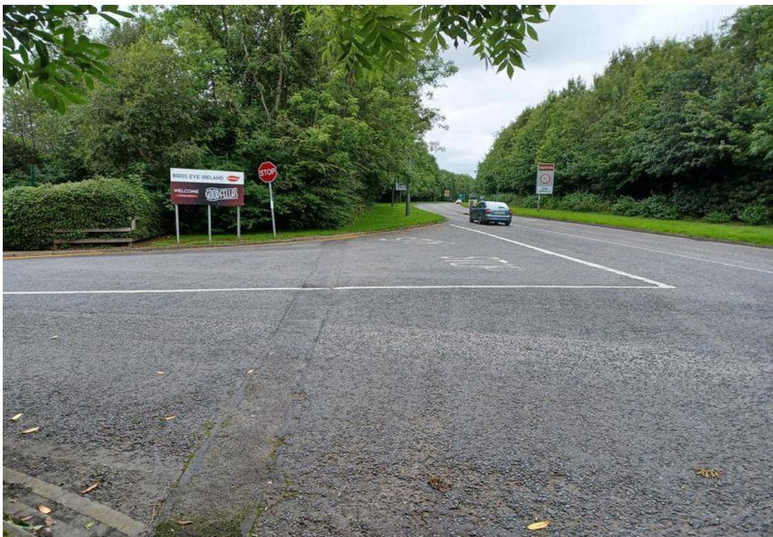
Image shows junction at entrance for Green Isle Foods. It is proposed to tighten this wide junction to a 9m radius.
