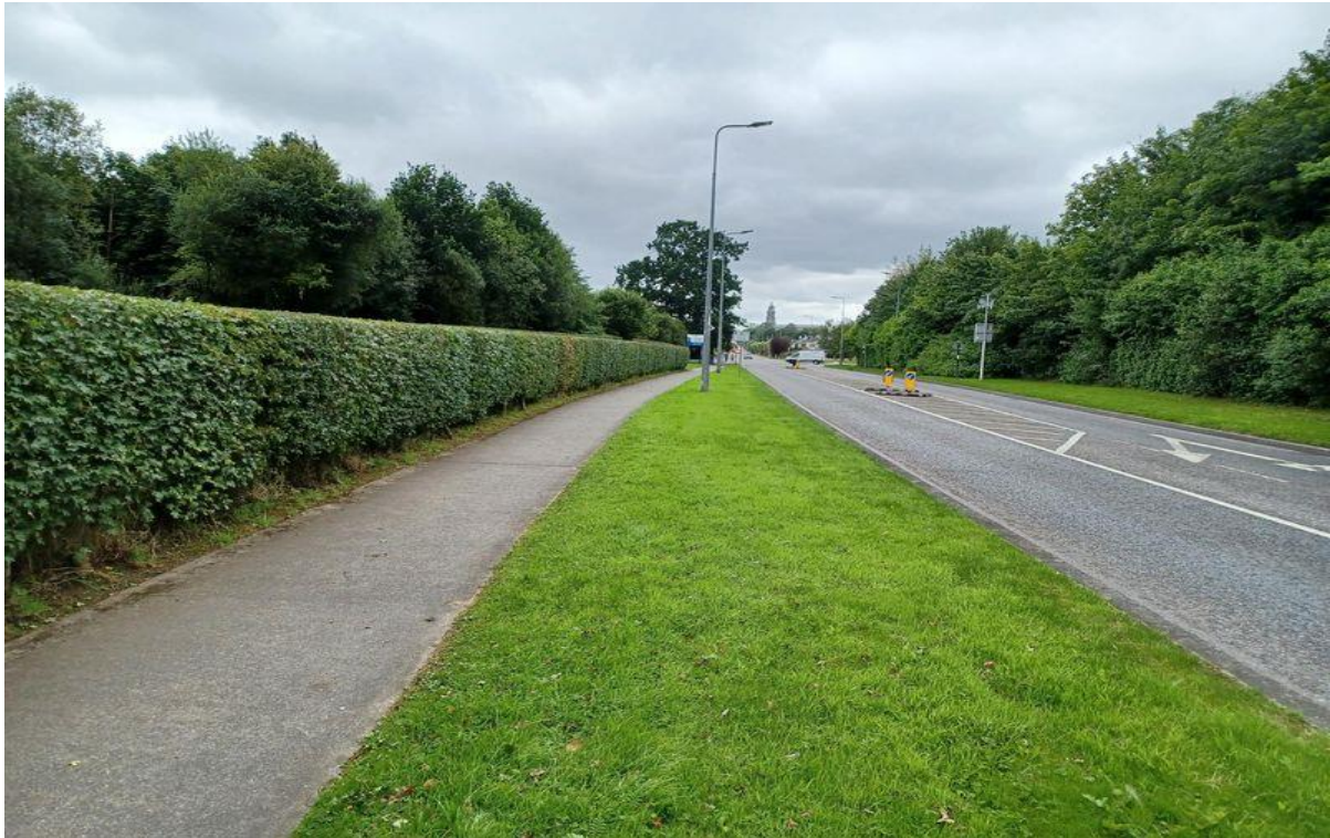
Image shows view towards Major Wells Road (Town Centre) from LHS with existing 2m path and Public Lighting columns.
