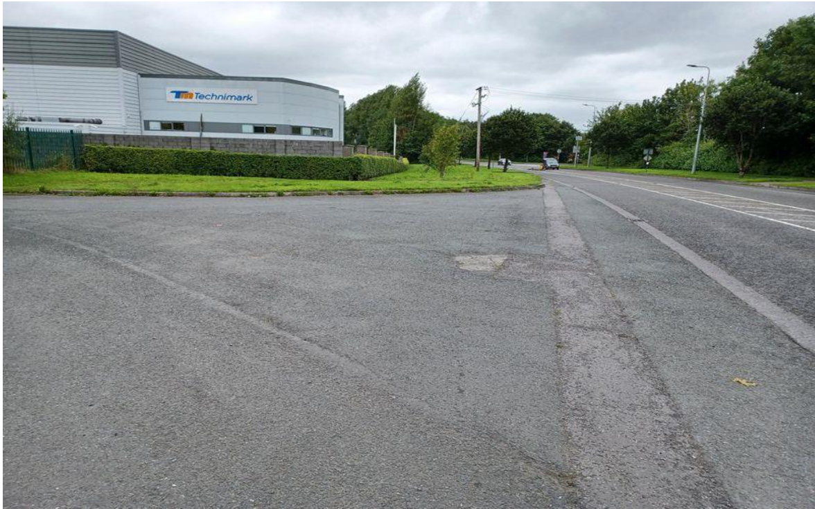
View at very wide junction at entrance to temporary Contractors compound. It is proposed to tighten this very wide junction to a 6m radius.
