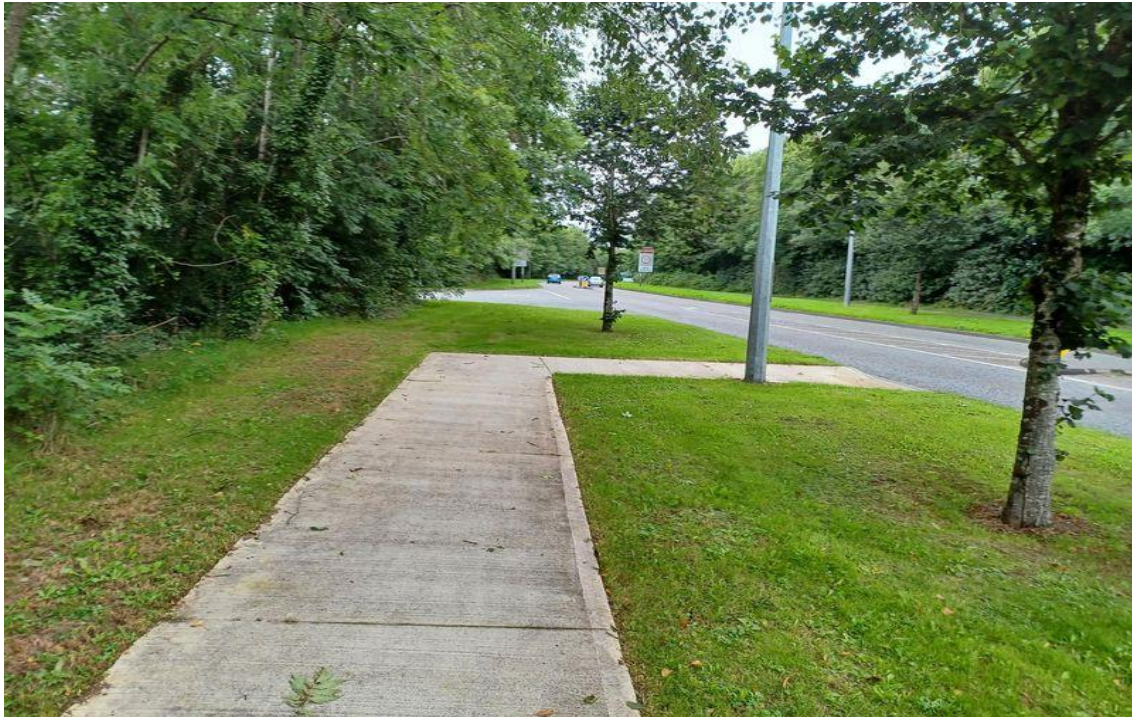
View of short length of existing path which serves the Business and Technology Park and crosses the N63 as shown.
