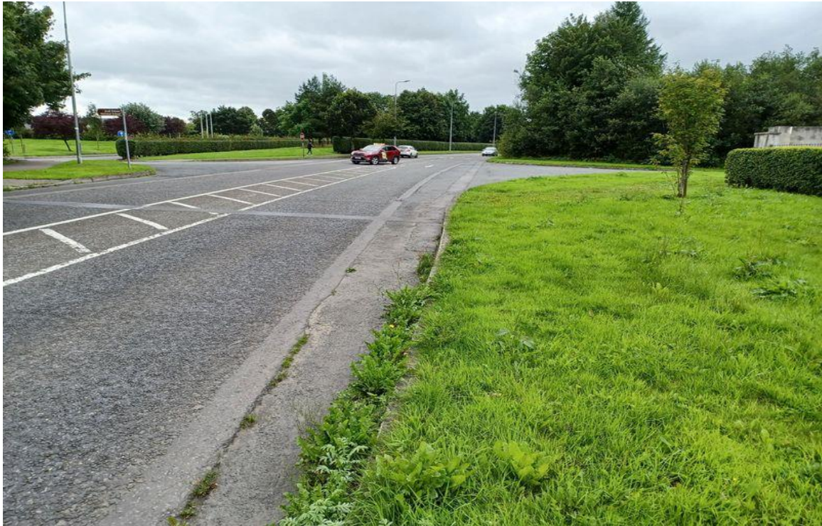
Image shows View towards Major Wells Road (Town Centre) from RHS @junctions. It is proposed to reinstate the old kerbline when Junction Tightening at this location.
