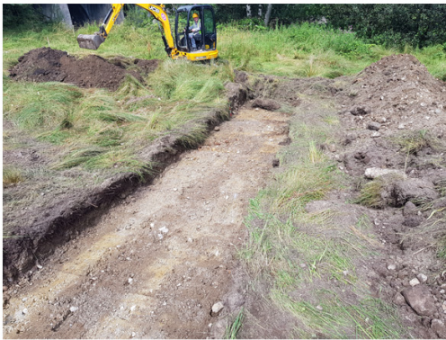
Plate 9: Trench 4. Eastern end. Looking SE. Scale 0.5m
