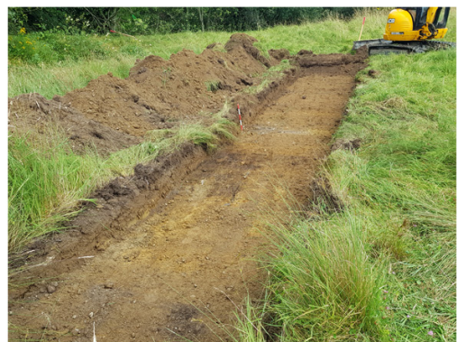
Plate 12: Trench 5. Looking N. Scale 0.5m. NB Trench 6 identical stratigraphy
