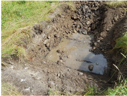
Plate 7: Trench 3. Showing made ground and water ingress. Looking N
