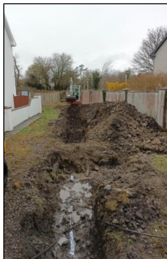
Plate 2: Looking north at excavation of test trench 2
