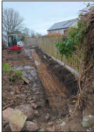
Plate 4: Test trench 1, looking north
