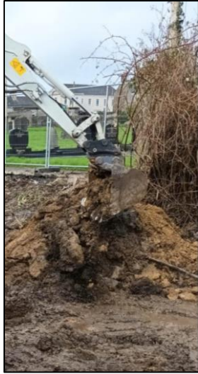
Plate 5: Demolition of the break in the existing stone wall
