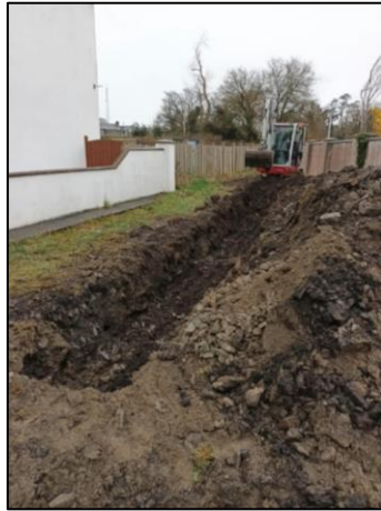
Plate 1: Looking north at excavation of test trench 2
