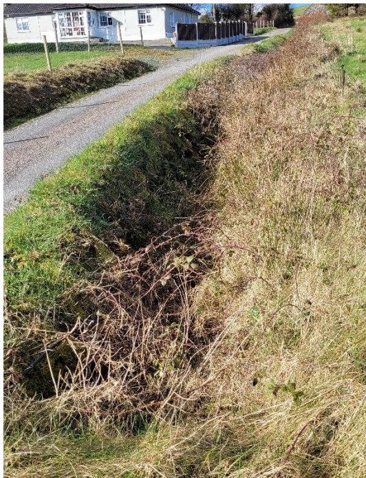
Image 4-1: Drainage ditch and earthbank on western boundary (northern-end) at roadside
