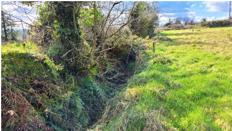
Image 4-4: Field margin at drainage ditch and earthbank on southern boundary.
