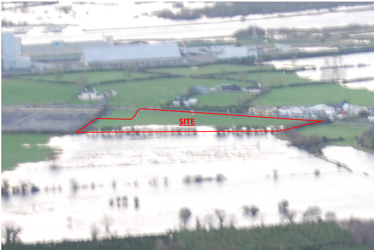
Photo 2: Flood Event November 2009
