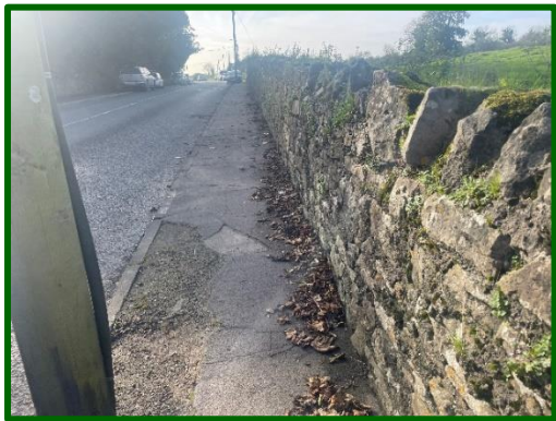
Picture 4: Stone walls and other stonework (BL1) on site
