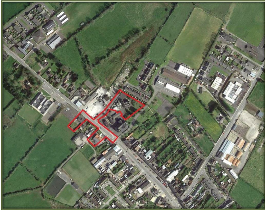
Figure 4 – Aerial Photograph of the Work Locations (Outlined in Red) and its Surrounding Habitats © Google
