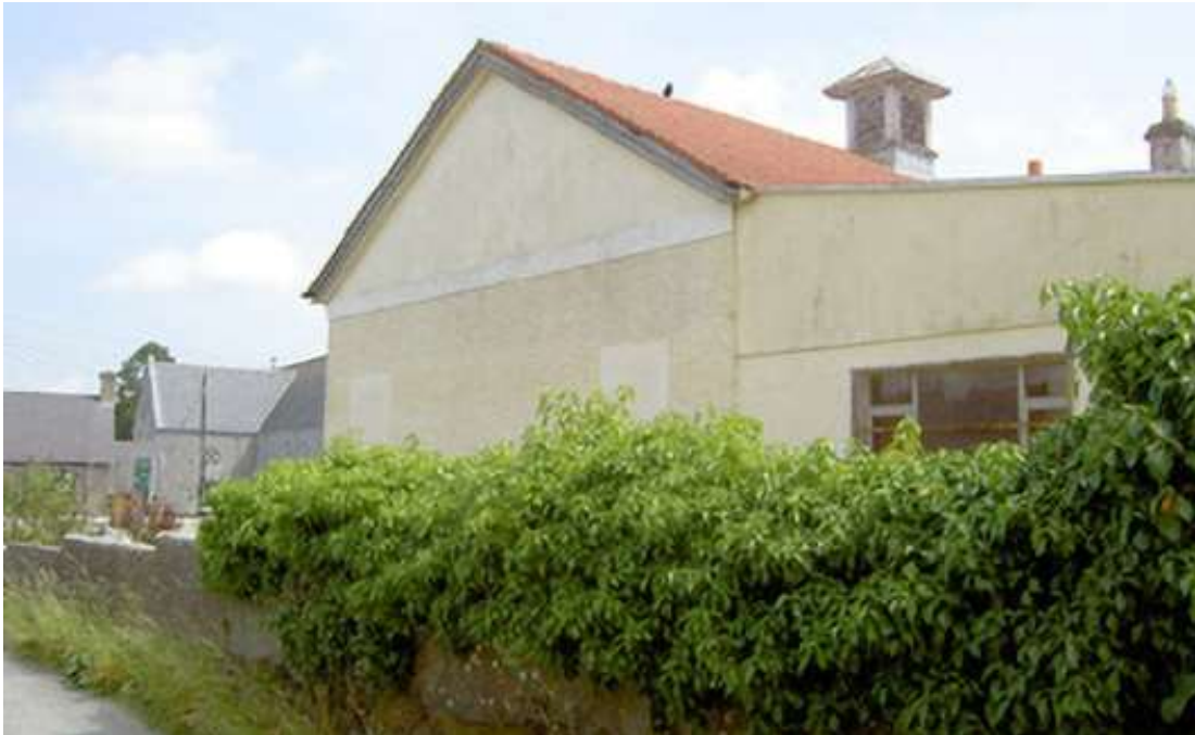
NIAH – Image of side elevation of Dean Egan Library c.2005 viewed from access road
