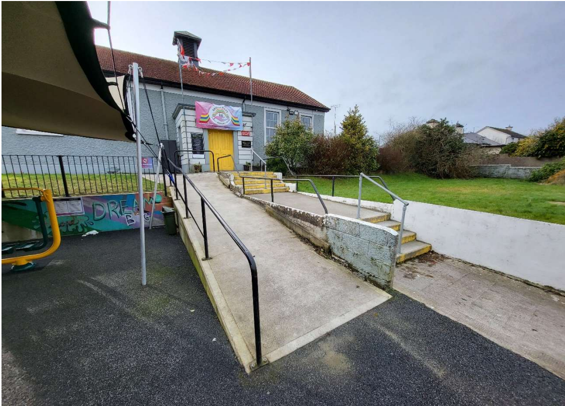
KLA – Image of the ramped approach to Dean Egan Library
