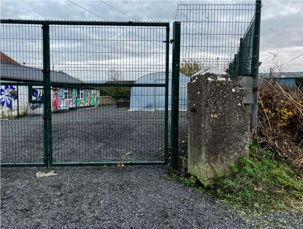
KLA – Image of existing extension and yard at the rear of the Dean Egan Library viewed from access road
