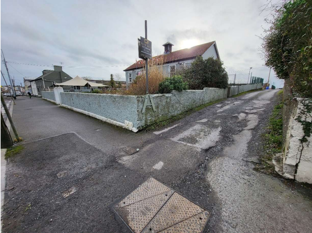
KLA – Image of the north-western corner of the Dean Egan Library and existing narrow access road
