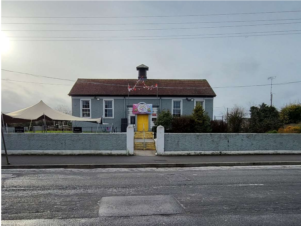
KLA – Image of the front elevation of the Dean Egan Library
