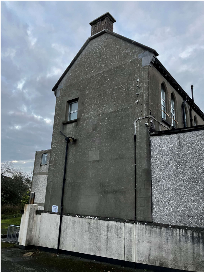
KLA – Image of protruding northern gable of Convent of Mercy
