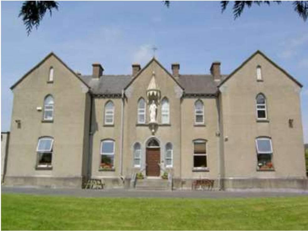
NIAH – Image of front elevation of the Convent of Mercy c.2005
