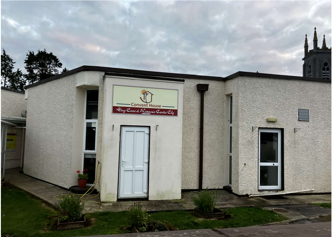
KLA – Image of hexagonal extension to be demolished viewed from northwest boundary
