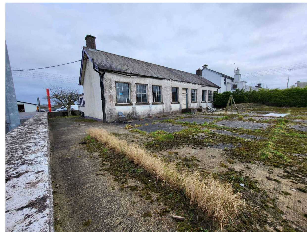
11. Schoolhouse rear elevation view.
