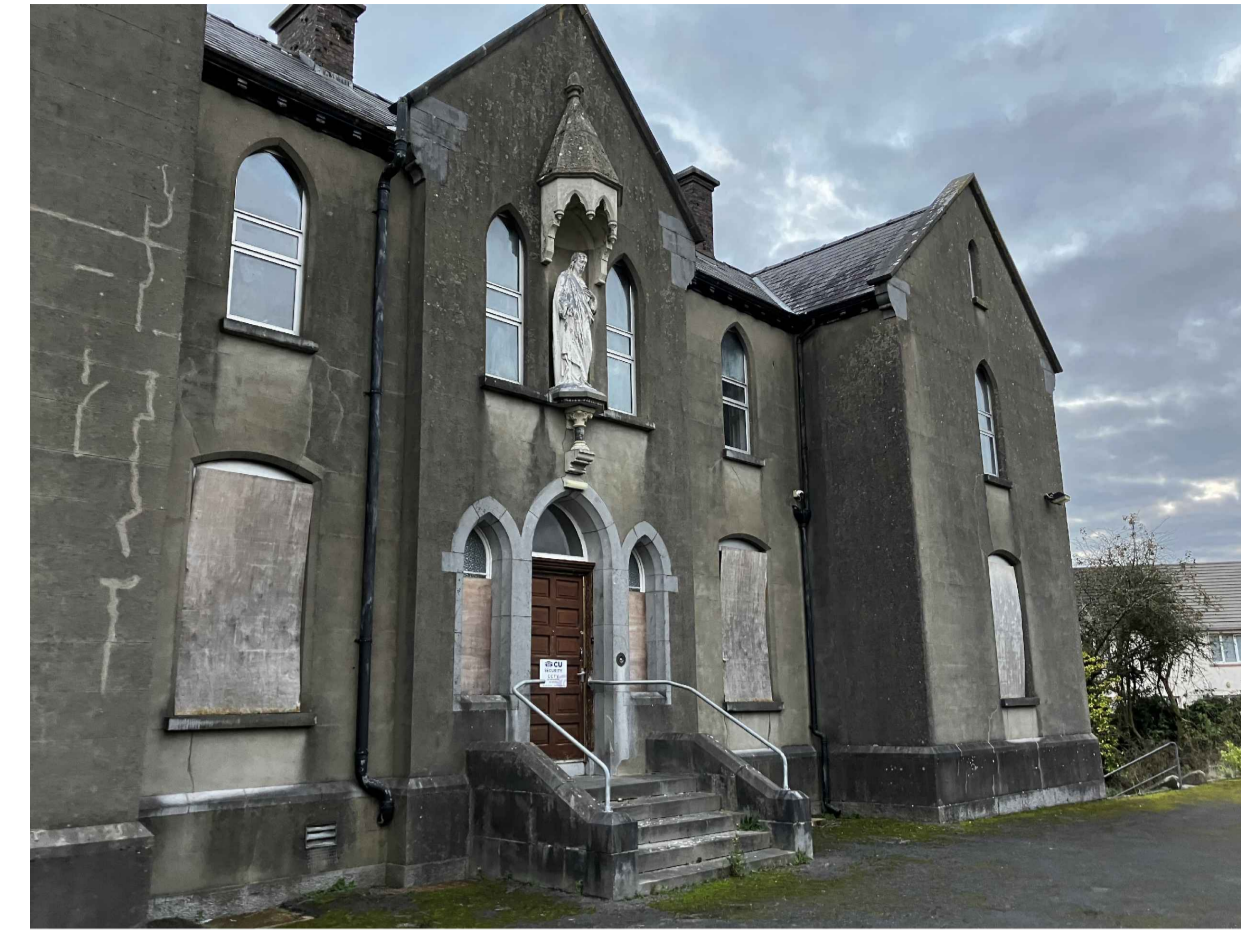
3. Convent of Mercy (Day Care Centre) front elevation view.
