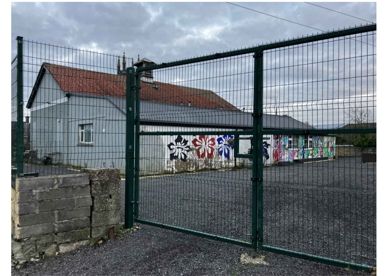
8. Dean Egan Library rear elevation view.
