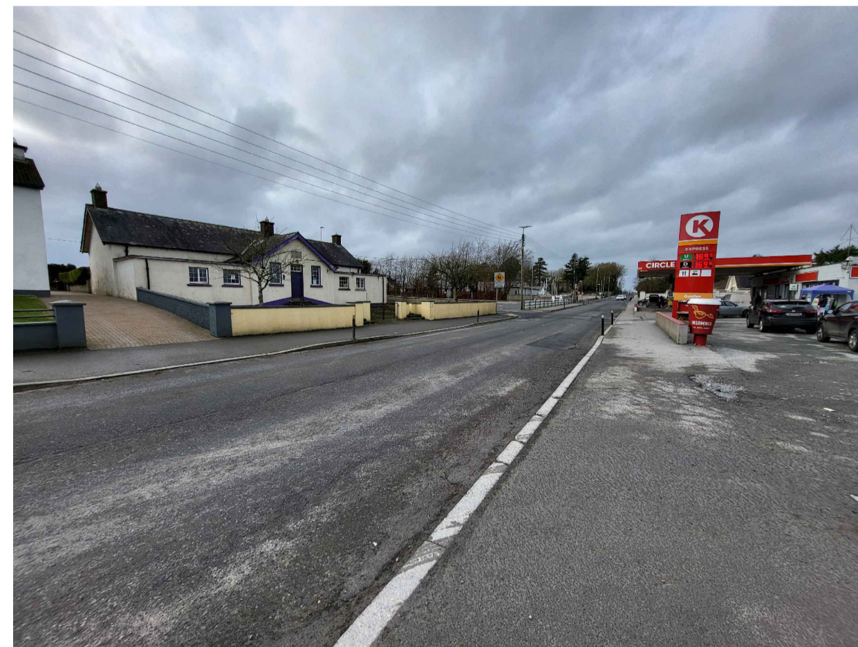
9. View of Schoolhouse from Main Street.
