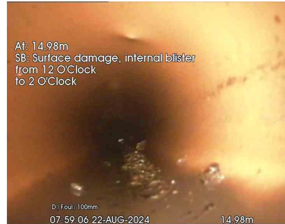
F1 TO F2_14-98m_075906.jpg, 00:01:10, 14.98 m Surface damage, internal blister from 12 o'clock to 2 o'clock
