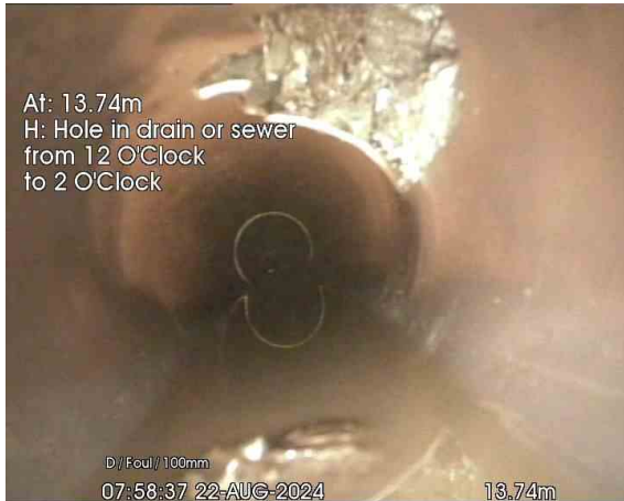
F1 TO F2_13-74m_075837.jpg, 00:00:53, 13.74 m Hole in drain or sewer from 12 o'clock to 2 o'clock
