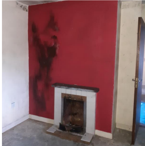
Internal photo showing smoke damage from chimney.
