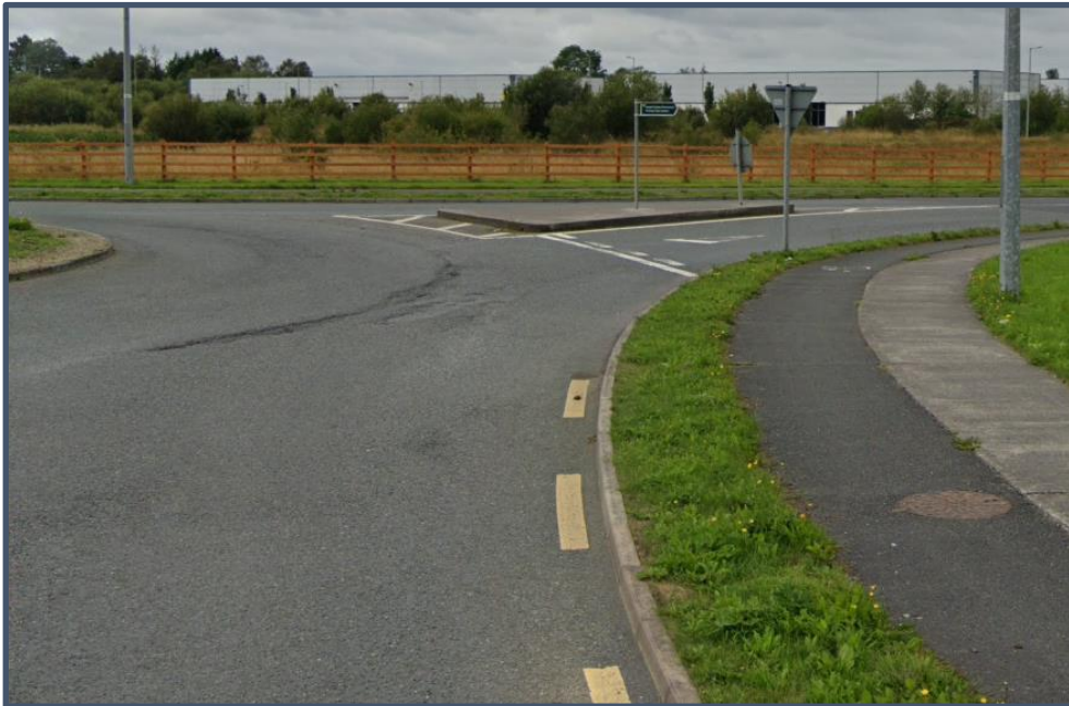
Figure 2-6 Facilities for non-motorised road users at Flancare Roundabout
