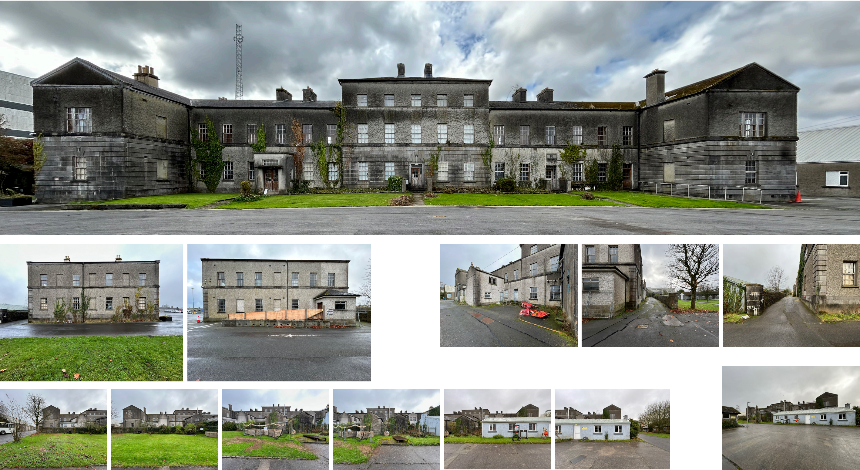
Selected exterior views of existing building. Complete photographic survey of exterior and interior is included within the accompanying Architectural Heritage Impact Assessment.
