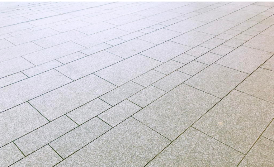
Natural stone paving combined with permeable mortar and bedding.
