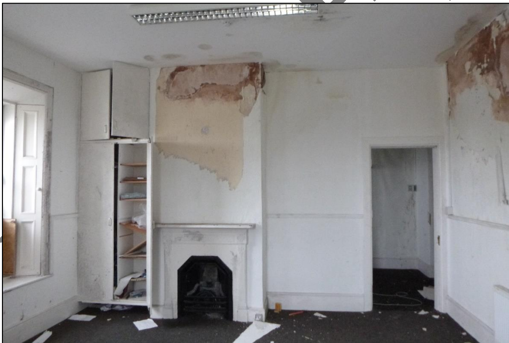
Plate 67 SW corner room to front range with chimneybreast and cast iron fireplace on internal NW wall (18.02.2025).
