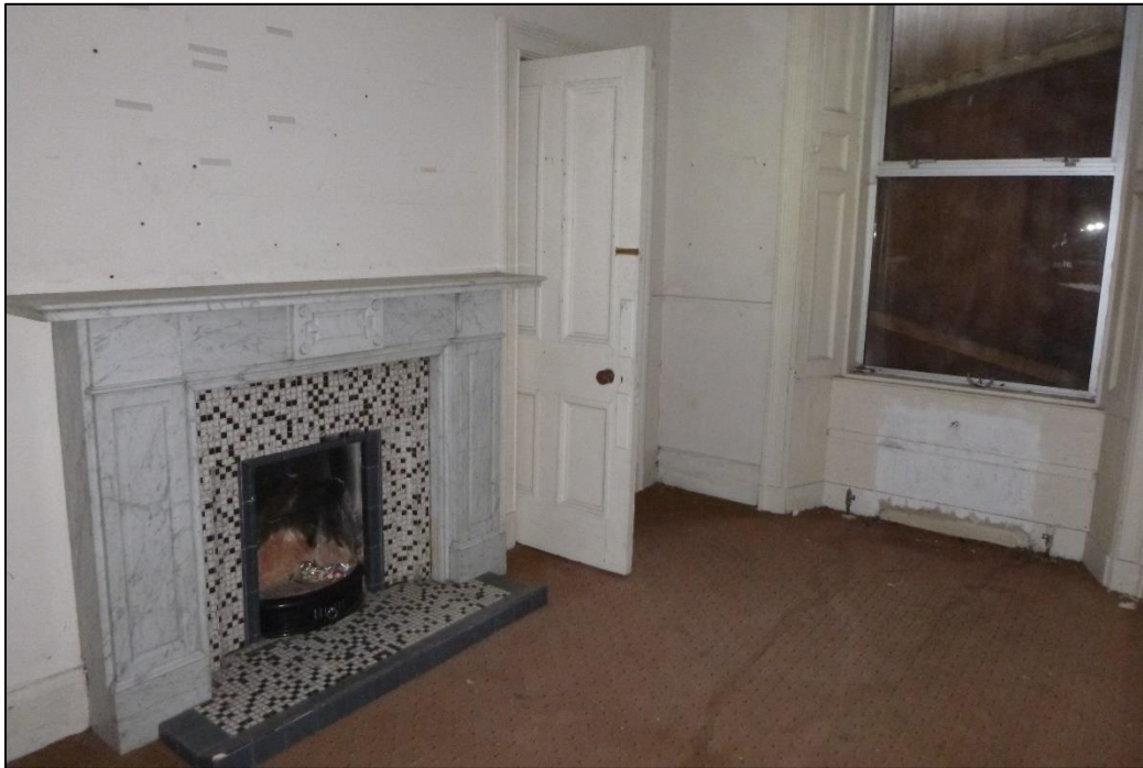
Plate 46 Small front parlour to SW side of front hall with timber 4-paneled door, fireplace and original shuttered window embrasure (18.02.2025).
