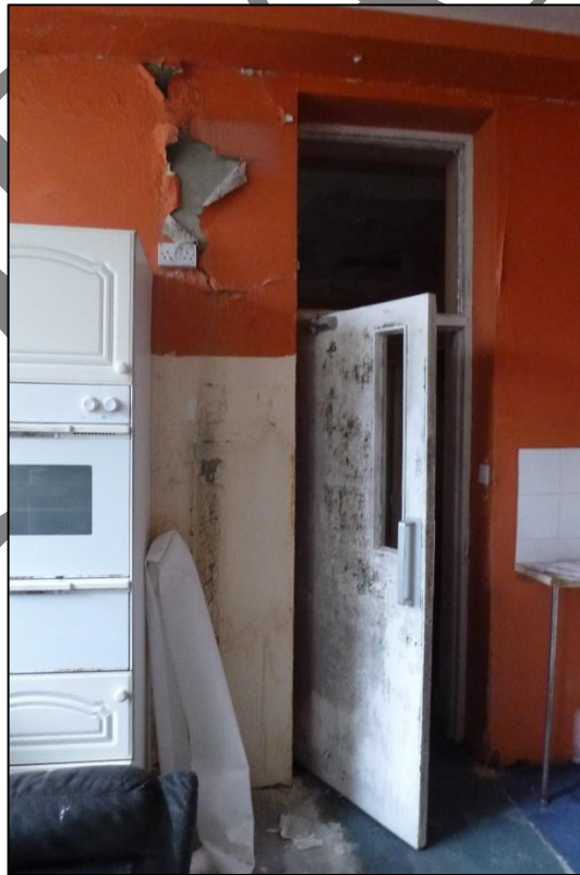
Plate 37 Ground floor annex kitchen with peeling paint on original SW external elevation and modified window opening at doorway (18.02.2025).
