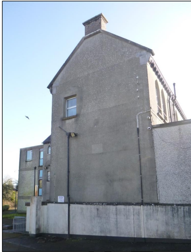
Plate 20 Rear NW gable end of SW range, with later window ope; painted wall at base continuing outside image to right beneath the modern annex is original to convent (05.02.2025).
