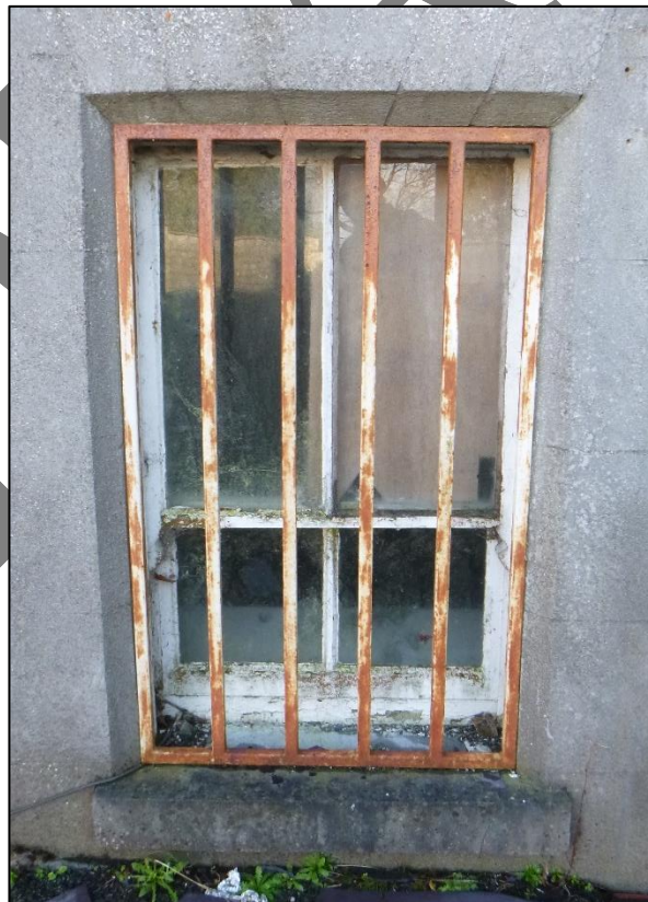
Plate 17 Close up of basement level timber sliding sash window on NW rear elevation of convent (05.02.2025).
