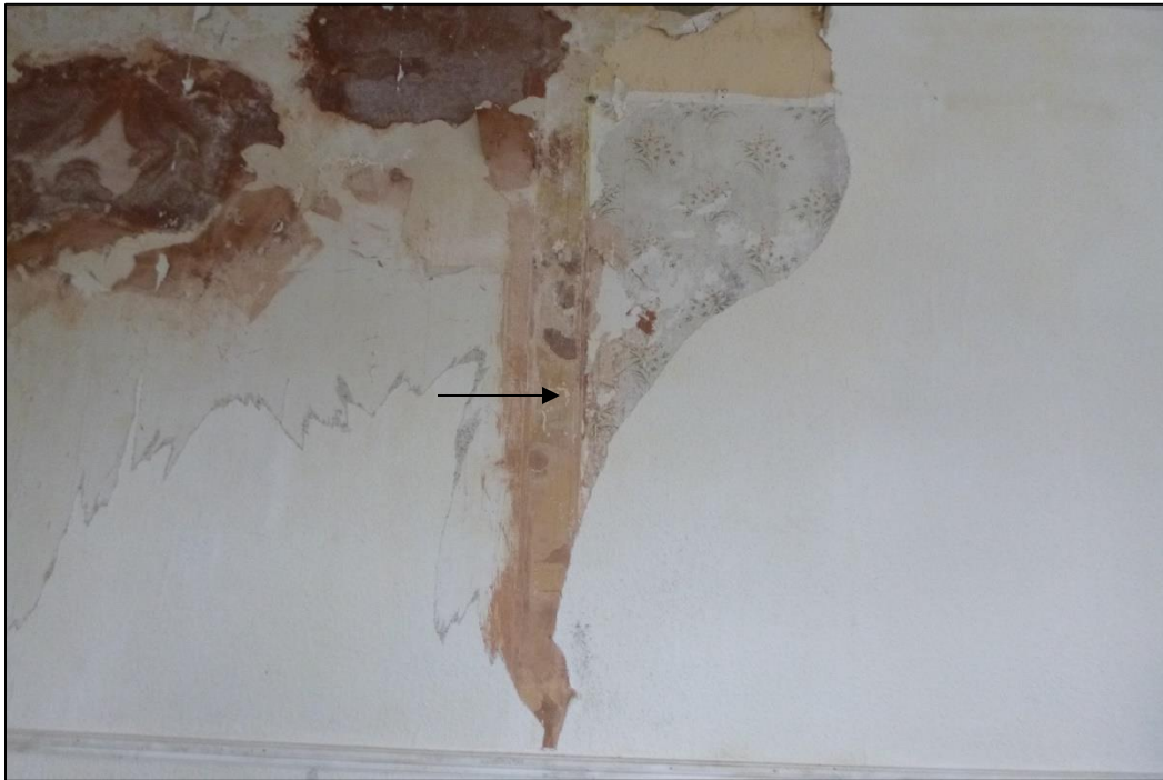
Plate 68 SW corner room to front range with early wallpaper and former partition scar (arrowed) on internal NE wall (18.02.2025).
