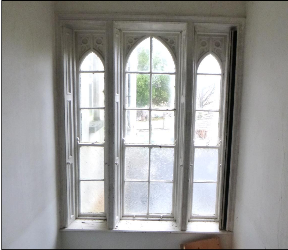
Plate 56 Tripartite window in NW elevation of rear range lighting stairwell at first floor level with original timber detail and decoration (18.02.2025).
