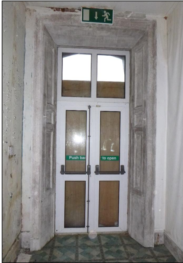
Plate 42 PVC fire escape at NE end of corridor with original timberwork internal to embrasure (18.02.2025).
