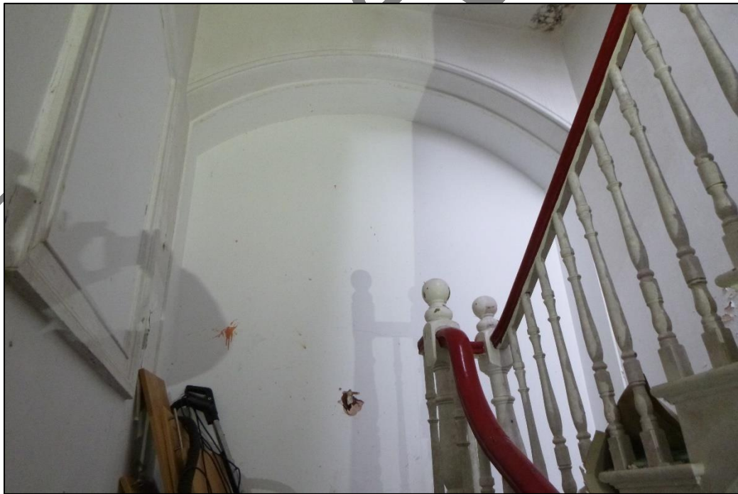
Plate 55 Stairwell landing at ground floor level showing blocked wide segmental arched ope (18.02.2025).
