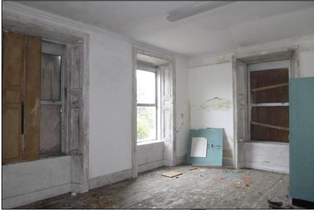
Plate 50 Community room at NE end of front range with original shuttered window embrasures, replacement aluminium window frames and timber floor (18.02.2025).
