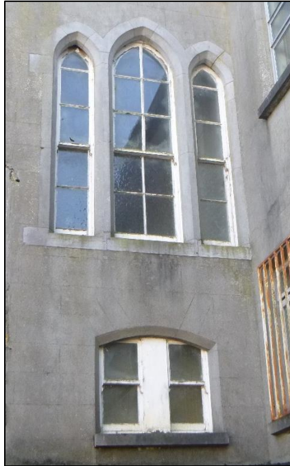
Plate 18 Timber sliding sash windows at stairwell on NW rear elevation of convent (05.02.2025).
