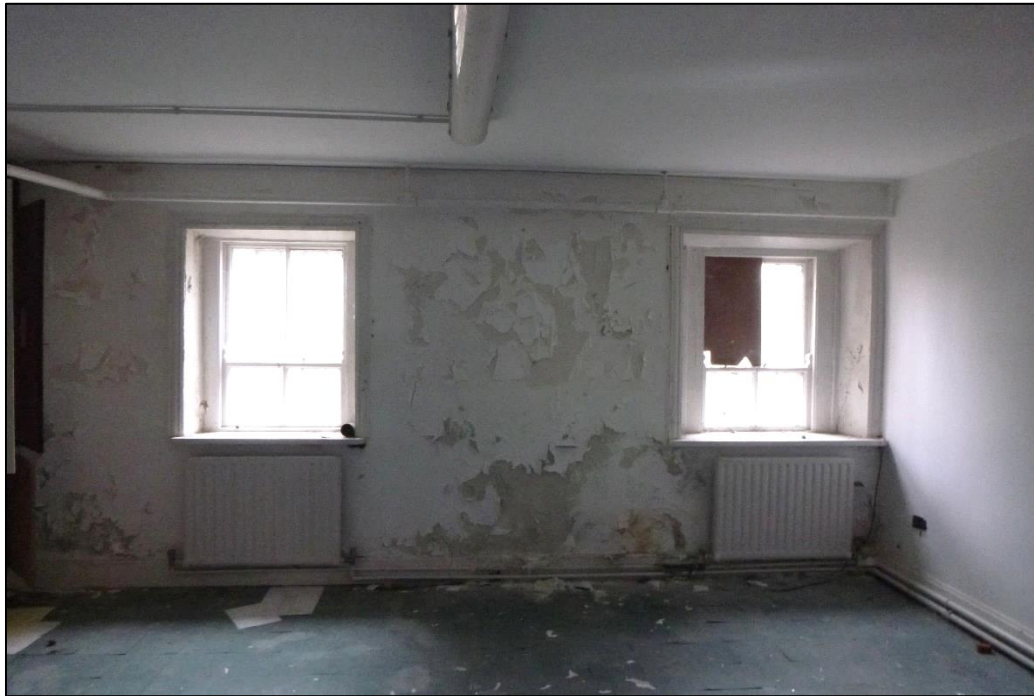
Plate 34 Basement room to SW end of rear range with original window opes and timber sash windows in NW elevation (18.02.2025).
