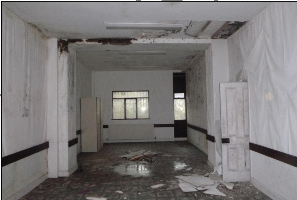
Plate 53 View NE from former refectory room to 20th century infill at NE corner of convent; original gable wall knocked through into extension (18.02.2025).
