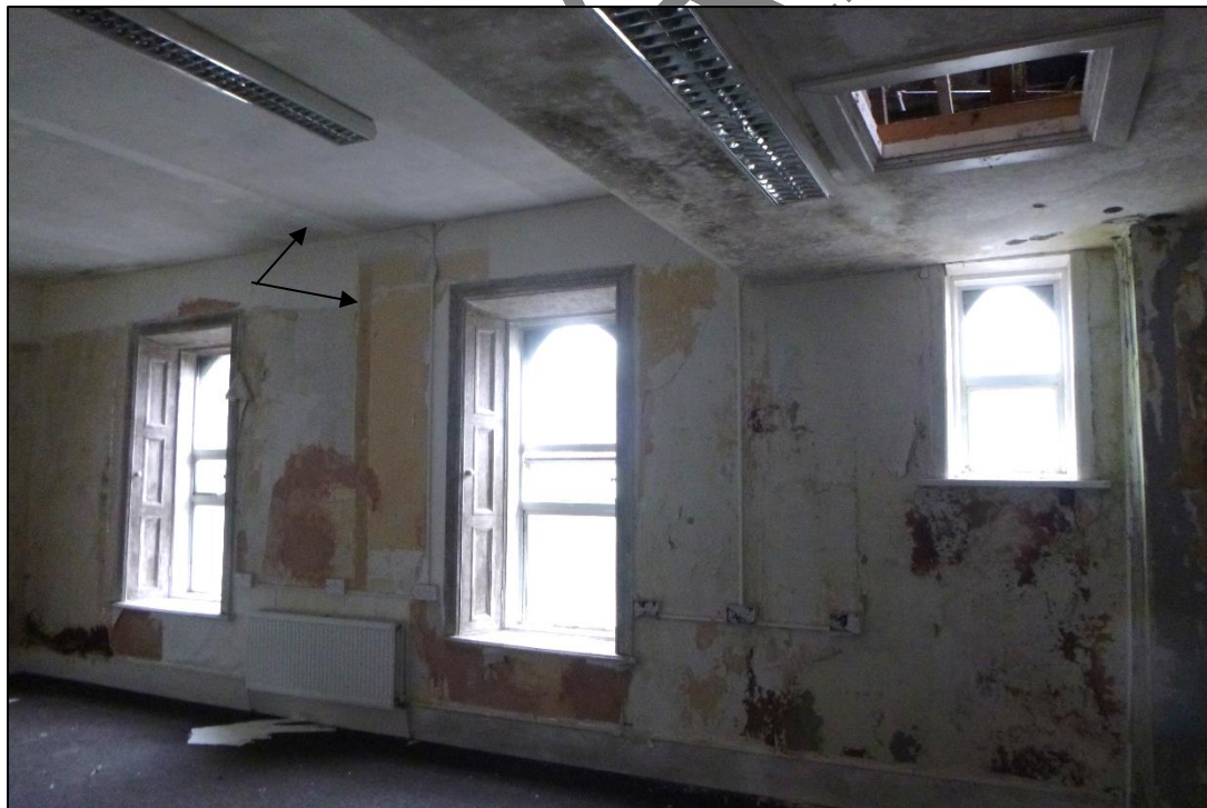
Plate 73 NW elevation of room to rear range, with lower ceiling and attic hatch above small window and partition scar (arrowed) (18.02.2025).
