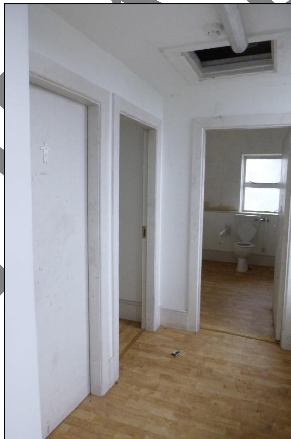
Plate 61 Later partition walls forming toilets in NW end of SW range, view to later window ope in NW gable (18.02.2025).
