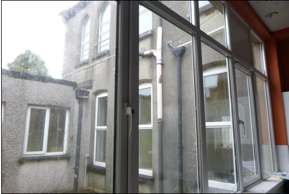
Plate 36 Segmental headed ground floor windows with PVC frames in SW elevation overlooking annex yard (18.02.2025).
