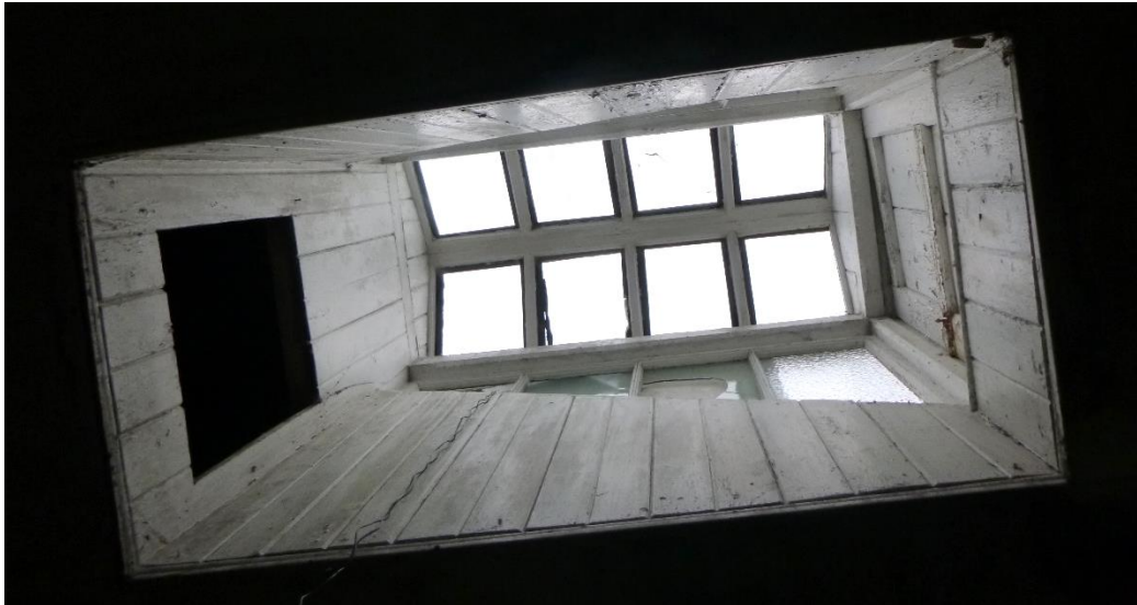
Plate 66 Timber roof light located centrally along first floor corridor (18.02.2025).
