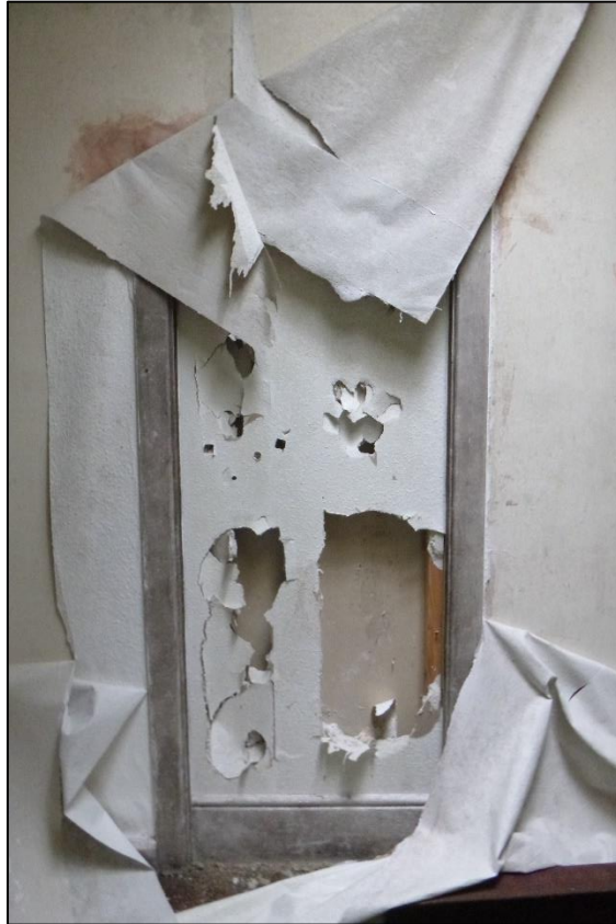
Plate 70 Blocked up door ope from corridor into former middle room in front range (18.02.2025).
