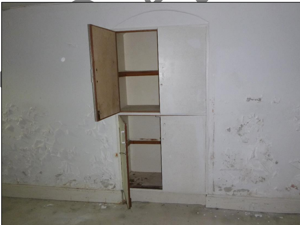
Plate 29 Infill cupboard in basement level corridor (SE wall) marking location of former segmental arched door opening (18.02.2025).
