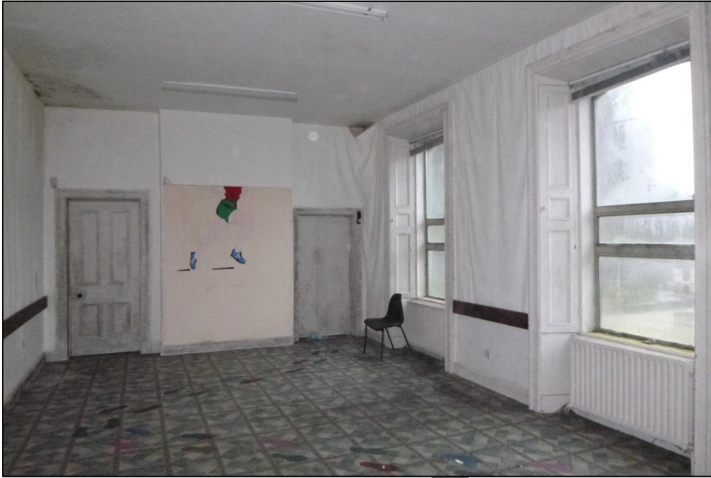
Plate 52 Former refectory room in rear range (view toward stairwell) with original shuttered window embrasures and replacement aluminium window frames on NW external elevation (18.02.2025).
