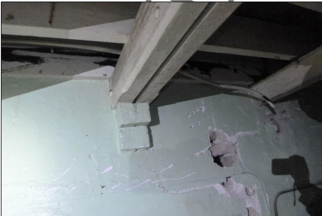
Plate 25 Original timber joists supported on brick corbels at basement level (18.02.2025).
