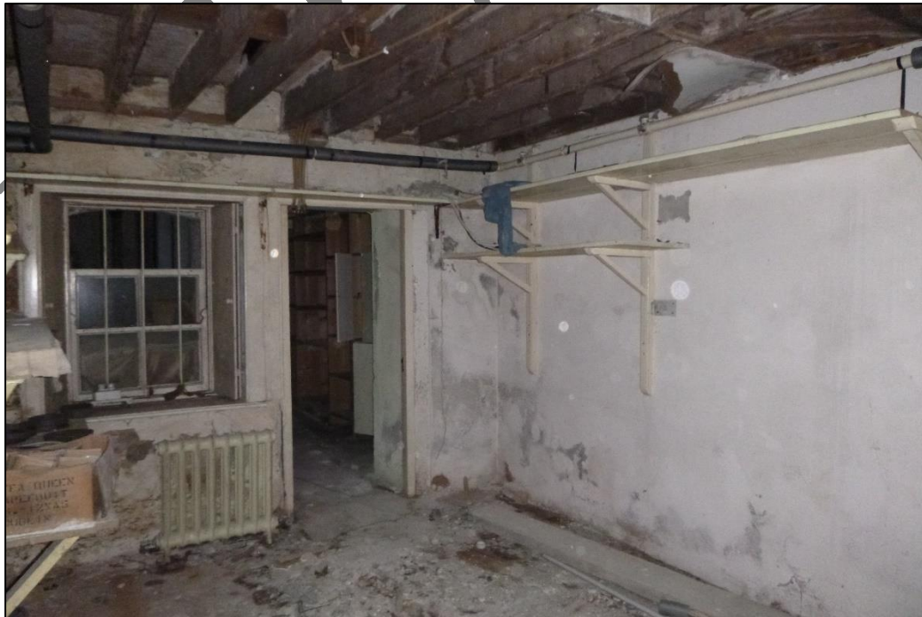
Plate 27 Basement level storeroom at NW end of SW range with original window ope and modified ope at door in original SW elevation; exposed joists above (18.02.2025).
