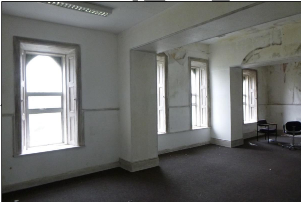
Plate 69 Enlarged central front room to front range with projecting stubs of original internal dividing walls, view to SW (18.02.2025).
