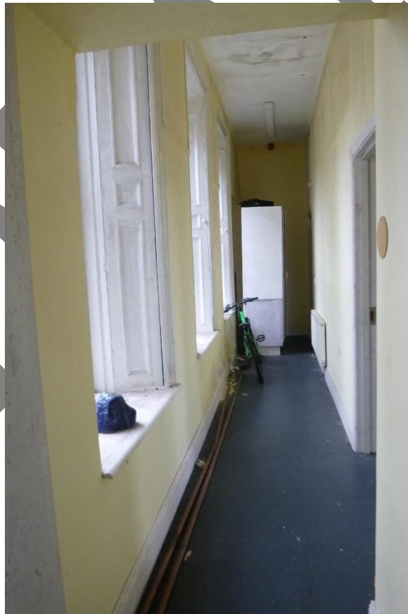
Plate 39 Ground floor corridor to NW corner of SW range with partition wall to right and original window opes with timber shutters to SW elevation to left (18.02.2025).
