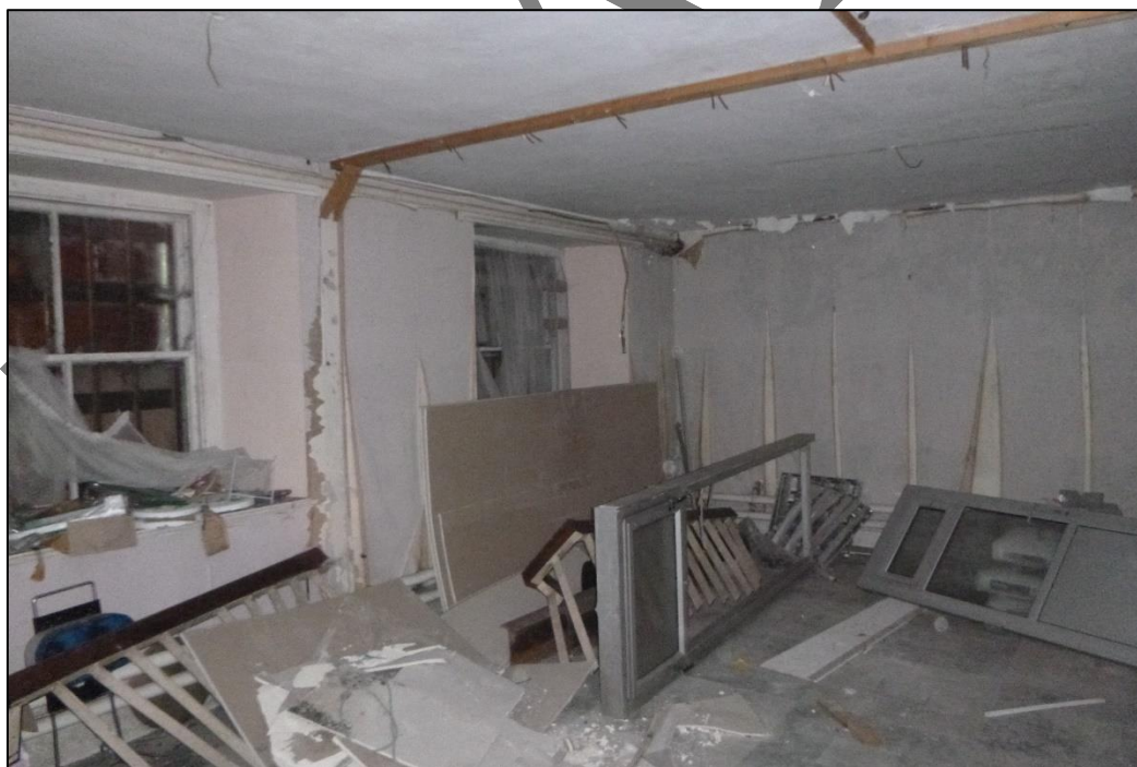
Plate 35 Basement level changing room to NE corner of front range with original window opes and timber sash windows in NE elevation; former room partitions demolished (18.02.2025).
