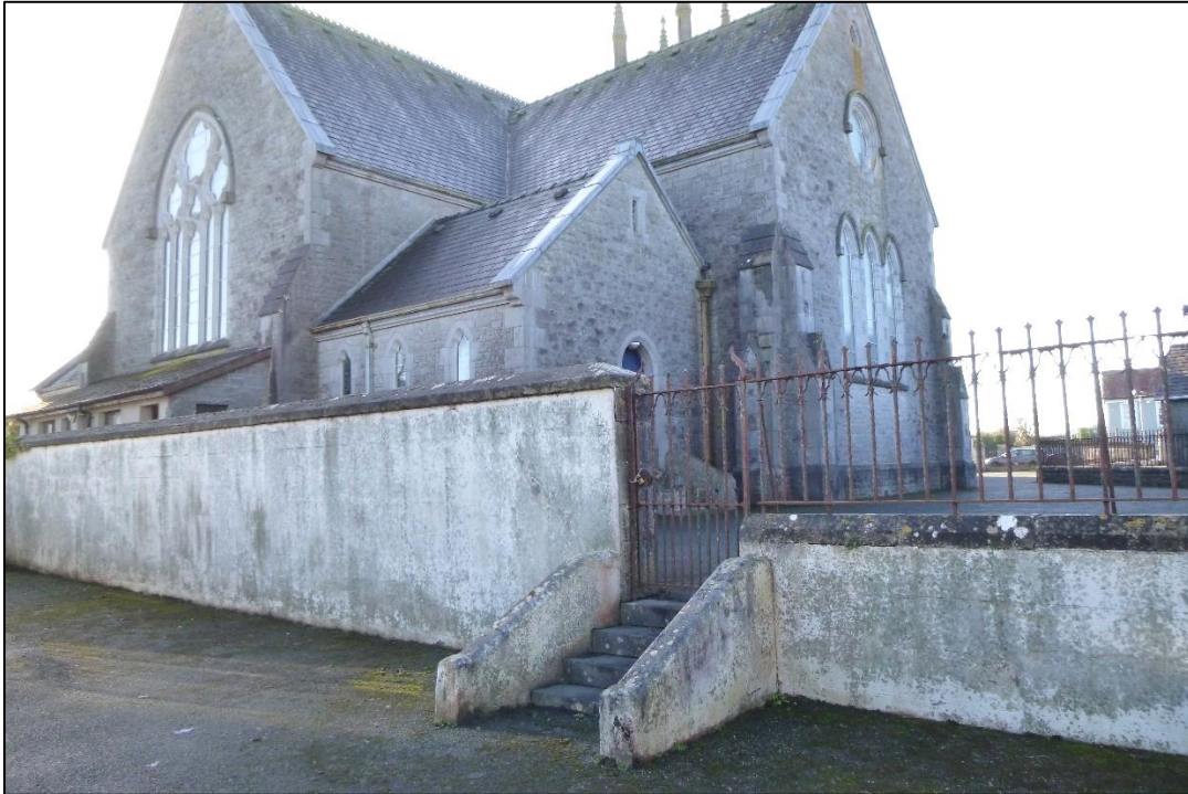
Plate 12 Cut stone steps with side walls from convent grounds into Saint Matthew's Catholic Church (05.02.2025).
