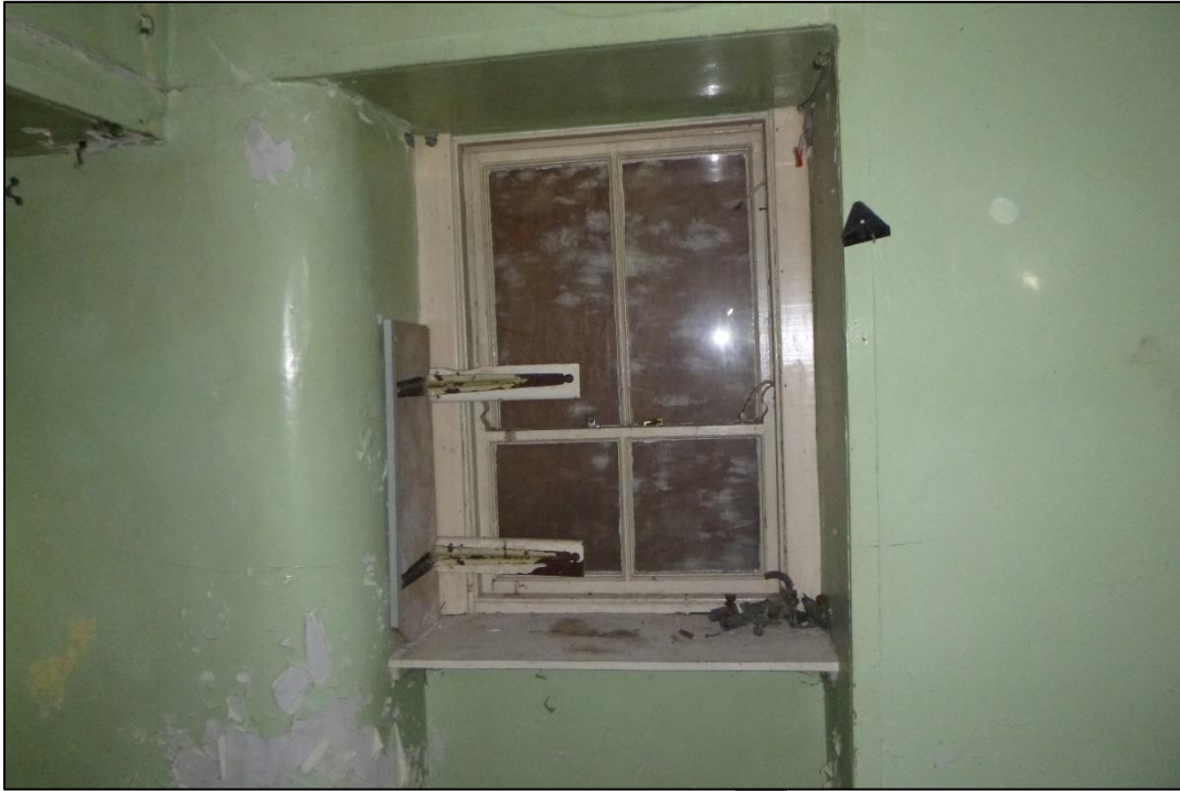
Plate 24 Blocked basement level window type with original timber sash window frame (18.02.2025).
