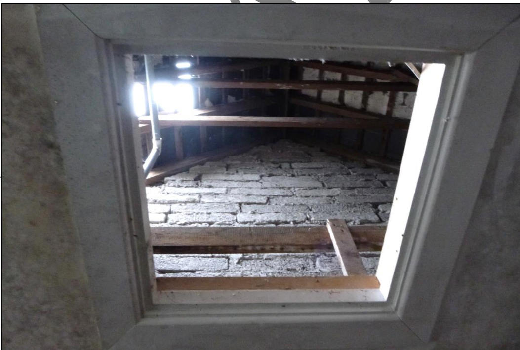
Plate 75 View through attic hatch to NE concrete block gable, original roof timbers and lime mortar torching (18.02.2025).
