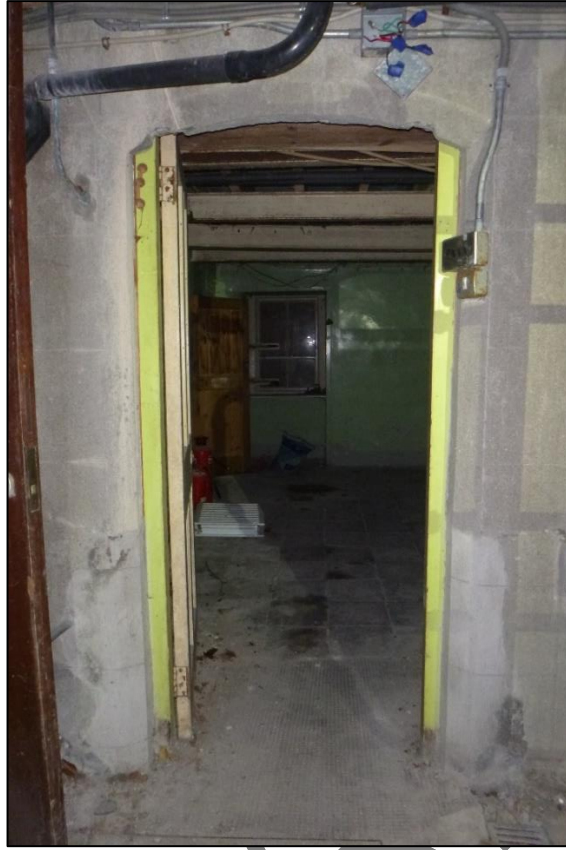
Plate 26 Sample modified window ope on SW elevation at basement level, accessing extended basement level to 1970s annex (18.02.2025).
