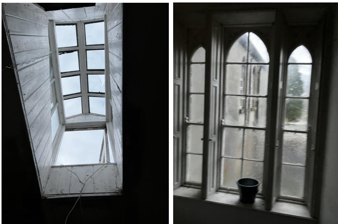
KLA – Image of original timber rooflights which are in severe disrepair & first floor feature window in the Convent of Mercy
