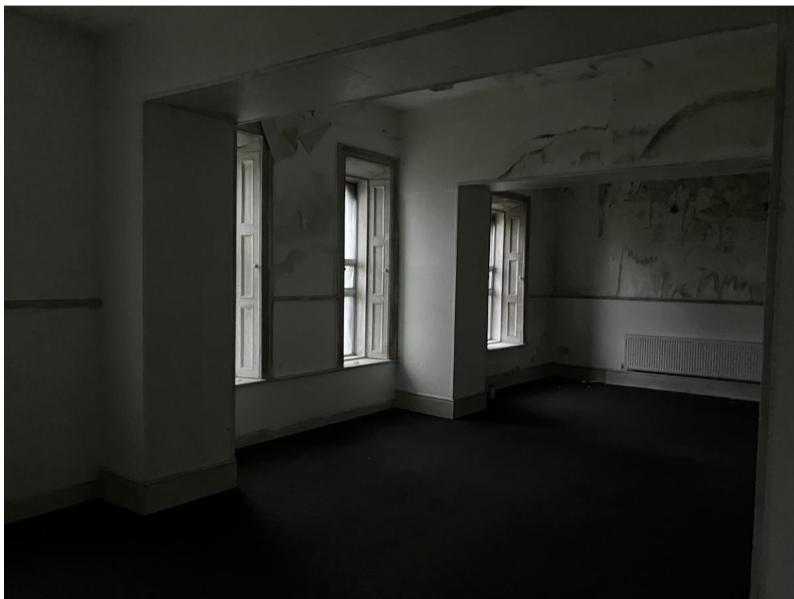
KLA– Image of the extensive water damage and damp on the upper floors
