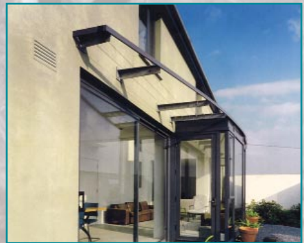
South façade of a house in Doolin, Co. Clare
