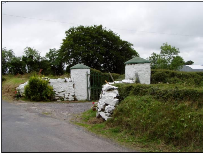
Whitewashed, barrel-style piers with stone wall splays on each side form an attractive entranceway commonly seen in rural areas.
