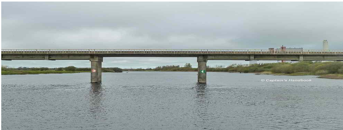
Pic. 9: Bord Na Móna bridge at Lanesboro.
