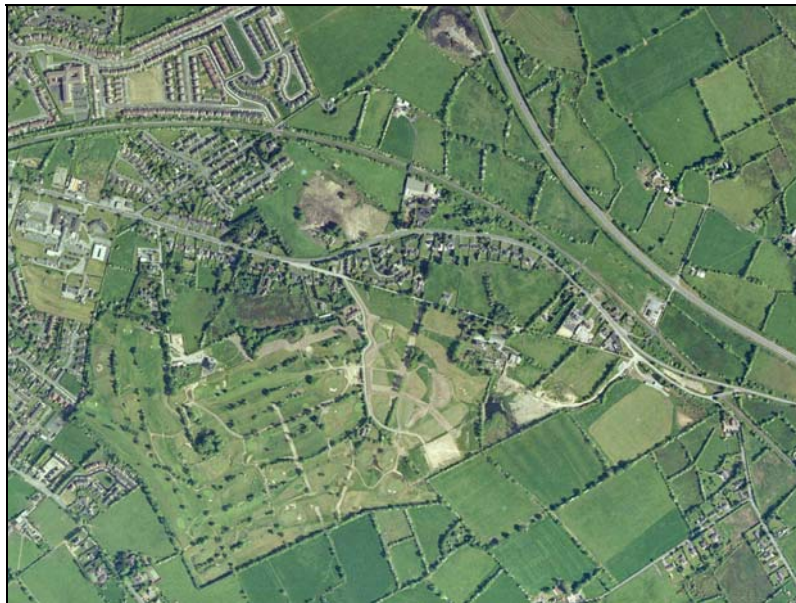
Arial photo of north eastern section of the LAP lands
