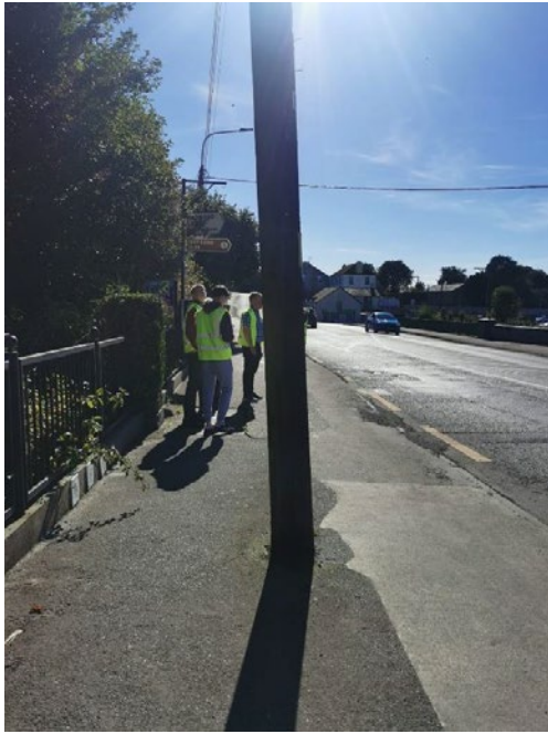
Pole in middle of footpath
