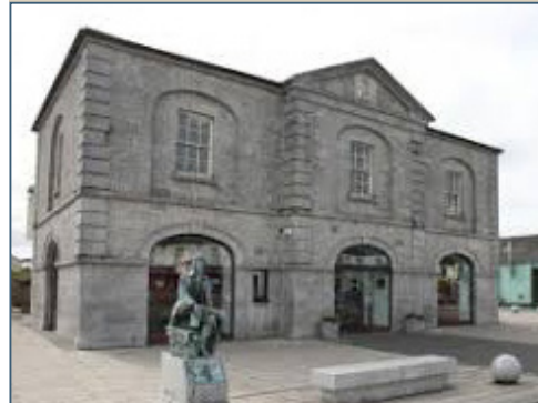
Fig.14 Courthouse & Market House, Ballymahon
