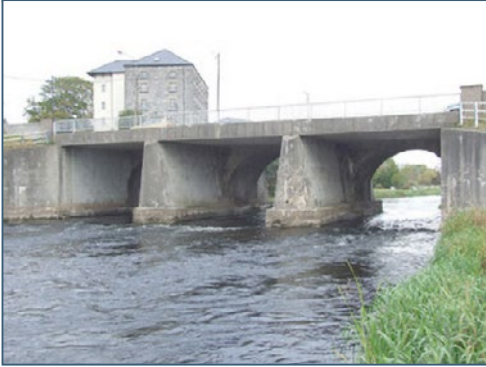
Fig.17 RIC Ballymahon Bridge, Ballymahon
