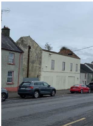
A building with no roof
