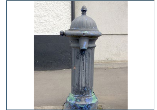
Fig.28 Water Pump, Ballymahon
