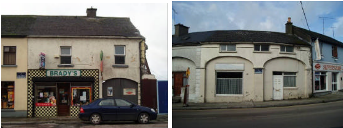
Areas of potential redevelopment within the town core. The buildings to the right contain interesting arch detail that should be retained on upgrading the area.
