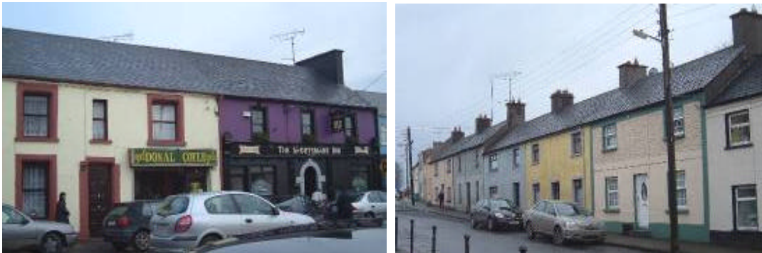
Terraces in main St (left) and Church St
