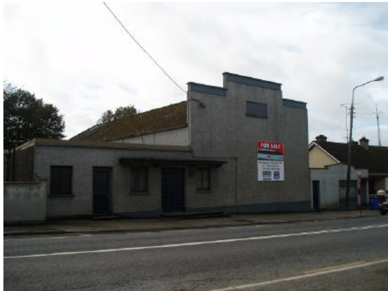
The site of the old community hall which is to make way for retail units.
