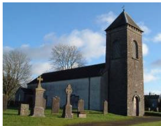
9. St. John's Church of Ireland Church
